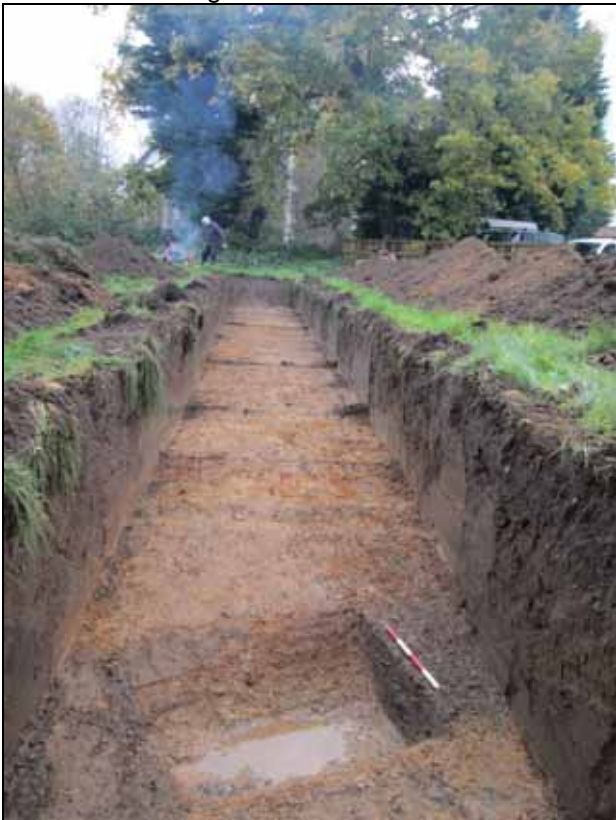
3 Post excavation shot of Trench 1
