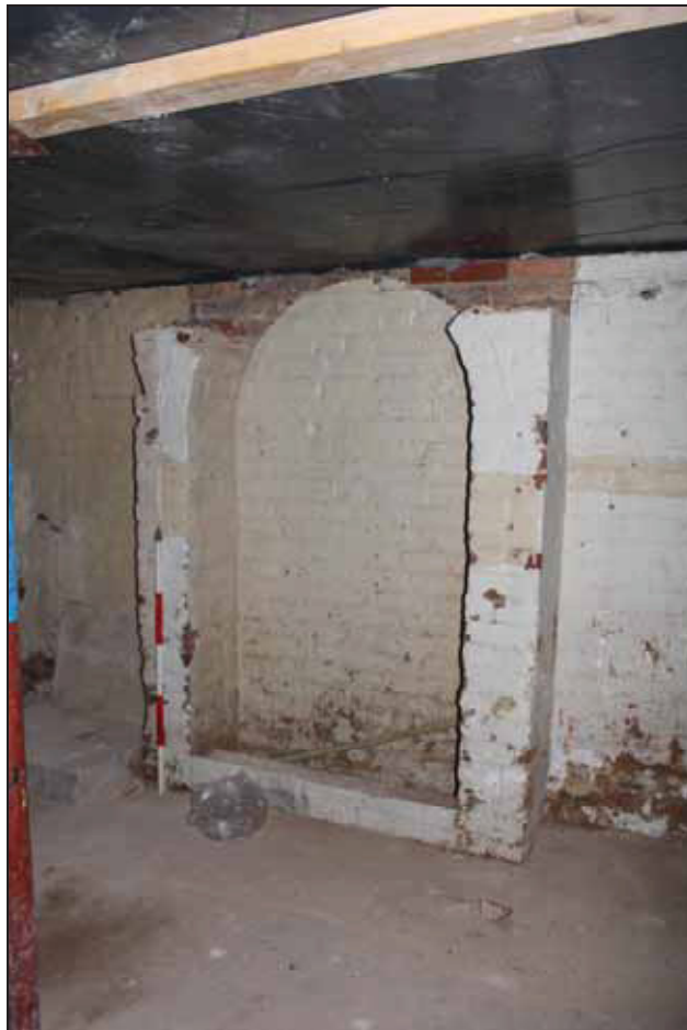
Plate 6: Base of former chimney stack on the east side of Room LGF04, taken from the south-west (DP 11)
