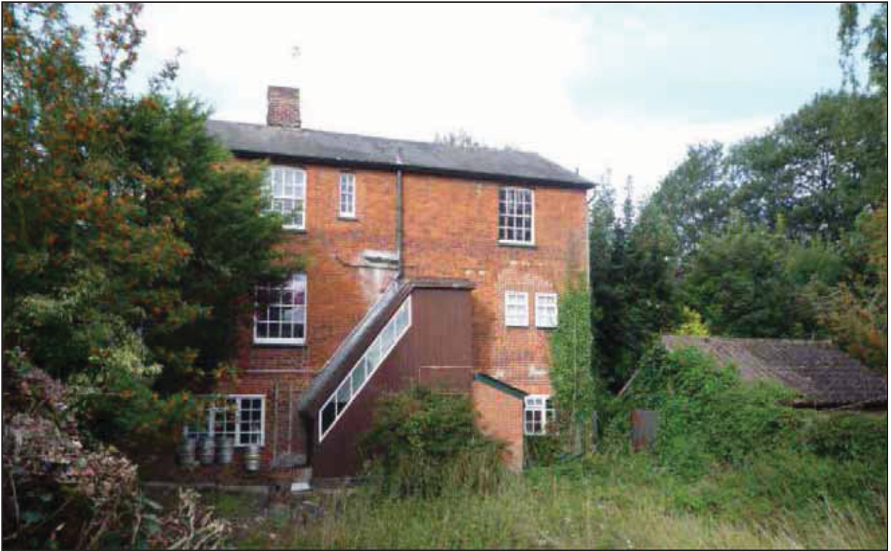
Plate 3: North-east elevation, taken from the east-north-east (DP 16)
