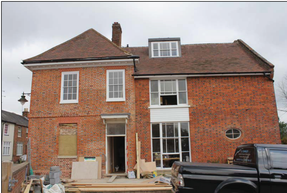
Plate 5 South elevation, taken from the south (DP77)
