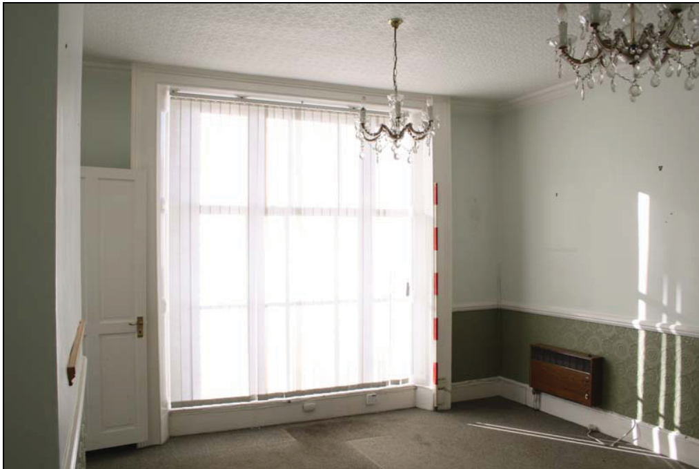
Plate 14 Large sash window, GF05, taken from the north (DP32)
