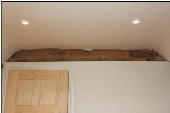
Collar retaining pegs for lower studs and upper roof structure, SF02, taken from the north-west
