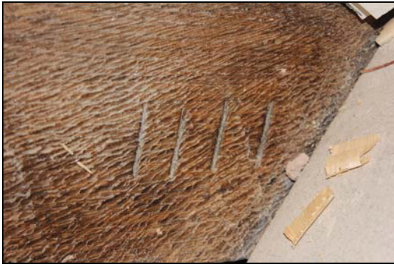
Assembly mark 'XX' to common-rafter, SF02, taken from the south-east
