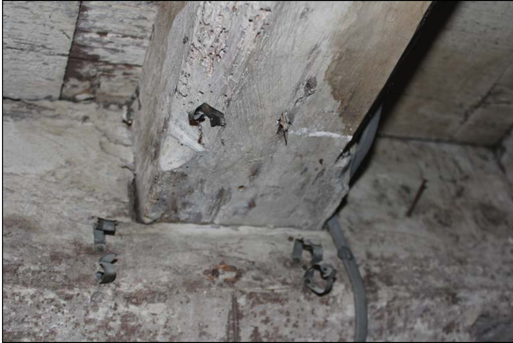
Plate 9 Lambs tongue chamfer stops to the common-joists, BF01, taken from the south-west (DP104)
