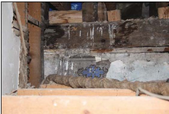
19 th century wall paper and plasterwork seen in the roof space above FF08, taken from the south-east
