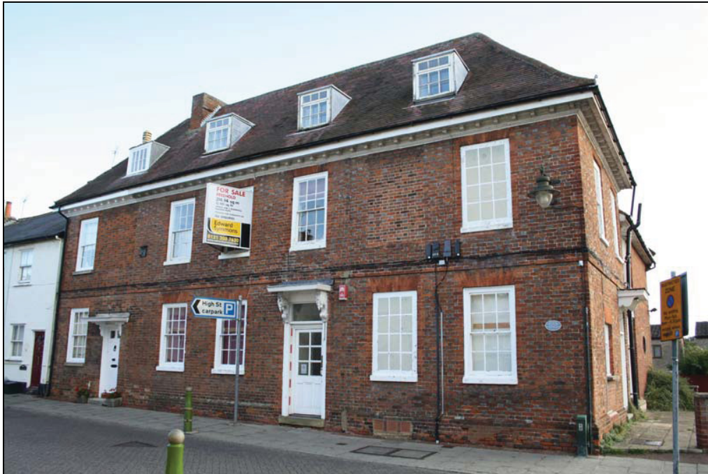
Plate 1 Main façade (west elevation), taken from the south (DP8)
