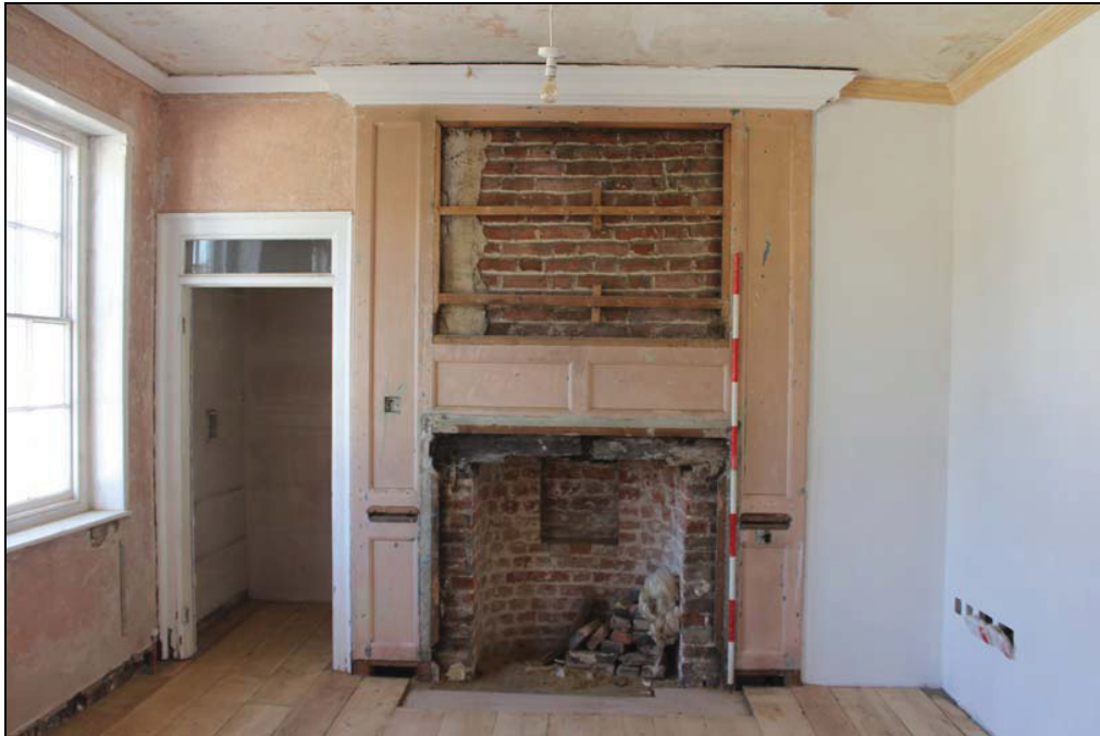
Plate 19 Exposed fireplace and surrounding panelling, FF02, taken from the south-east (DP110)
