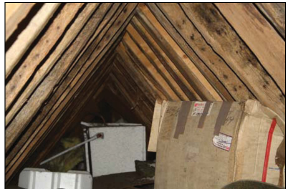
Rafter couples rising above collar level, taken from the north-west
