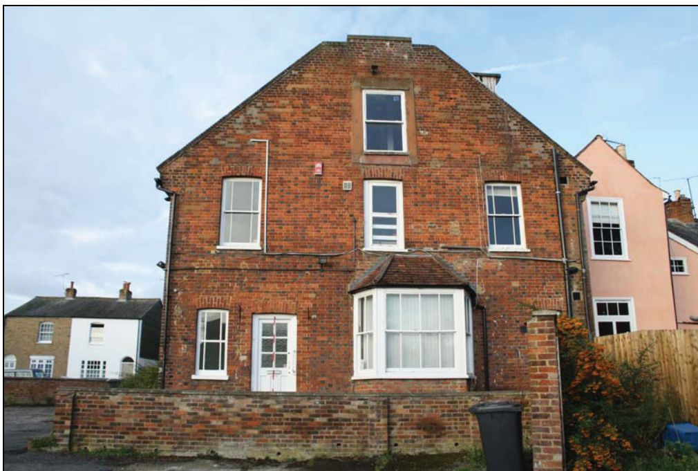
Plate 6 East elevation, taken from the north-east (DP7)
