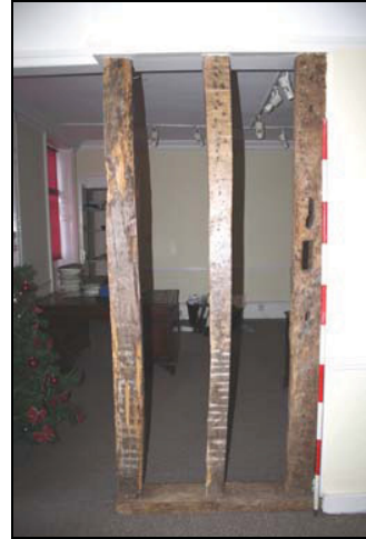
Studwork partition with re-used members, GF01, taken from the south-east
