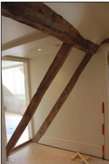
Assembly mark 'IIII' to common-rafter, SF02, taken from the south-west
