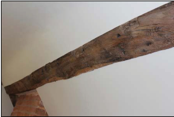
Eastern purlin with peg holes for rafters above and below, SF03, taken from the south
