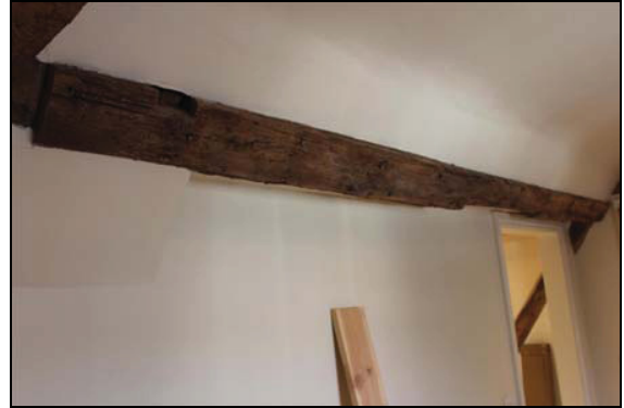
Eastern purlin with regular arrangement of pegs for common-rafters above and below, SF04, taken from the north-west
