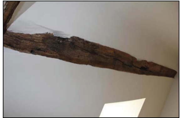
Western purlin with peg holes for rafters above and below, SF03, taken from the south-east
