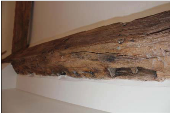
Western purlin with regular arrangement of pegs for common-rafters above and below, SF04, taken from the north
