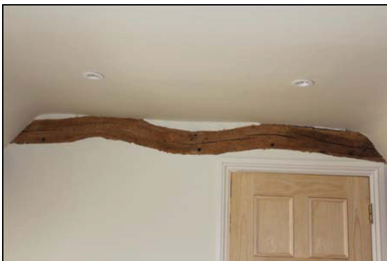
Waney collar at the bay division with peg holes for studwork, SF03, taken from the south
