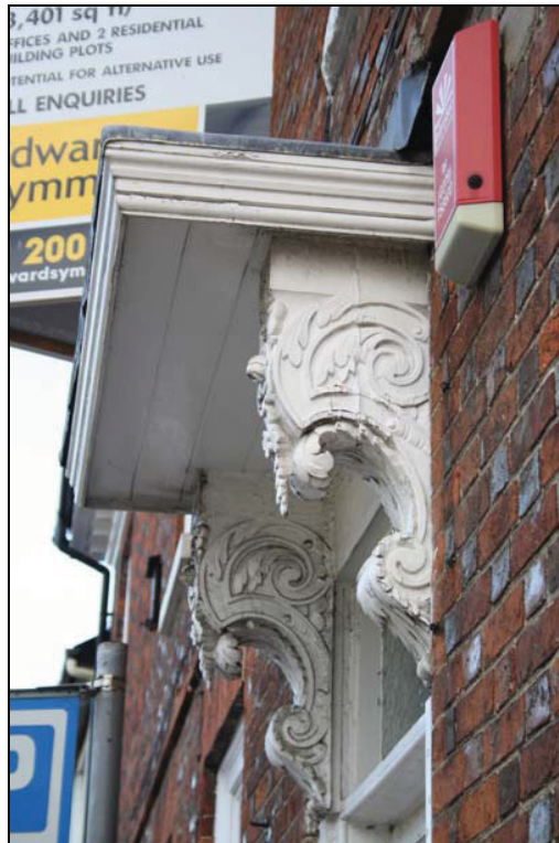
Plate 3 Detail of the decorative scrolled brackets supporting the hood above the main entrance, west elevation, taken from the south (DP11)
