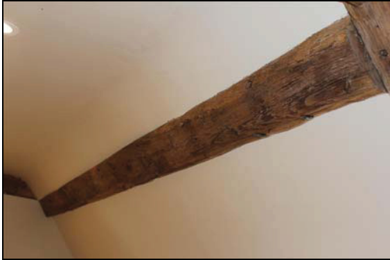
Western purlin with regular arrangement of pegs for common-rafters above and below, SF04, taken from the north
