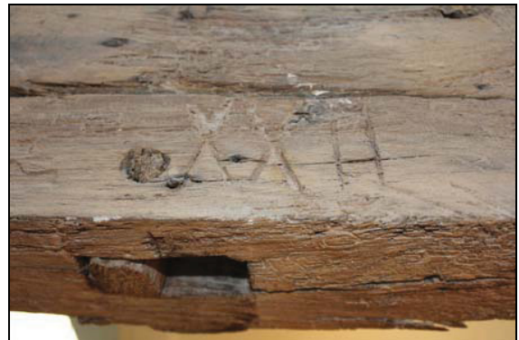
Assembly mark 'XXII' to purlin at junction with common-rafter now removed, SF02, taken from the north-east
