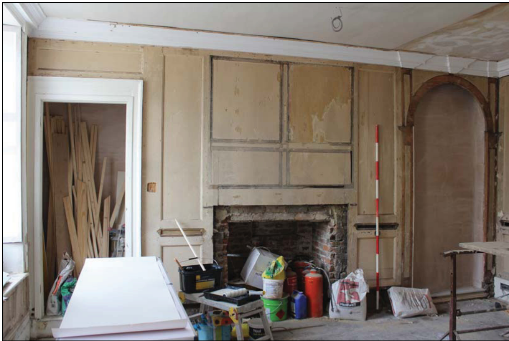
Plate 12 18 th Century wall panelling surrounding fireplace, northern wall, GF02, taken from the south-west (DP80)
