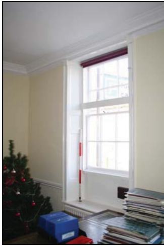
Sash window with splayed reveals, GF02, taken from the north
