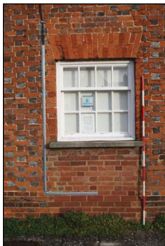
Window with disturbed brickwork below, south elevation, taken from the south-east
