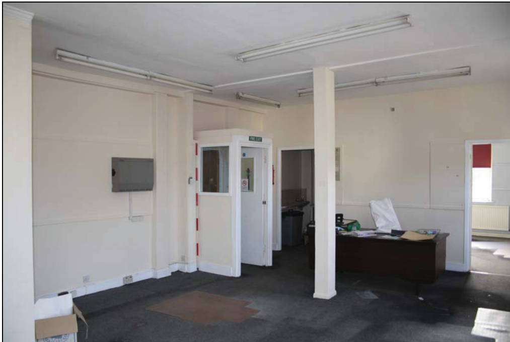
Plate 18 FF02, taken from the west (DP53)
