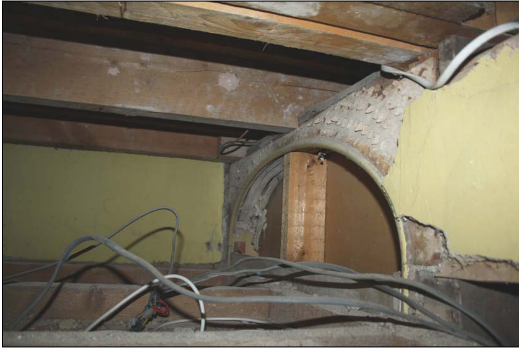
Plate 21 Arch concealed within in the roof space above FF08, taken from the north (DP60)
