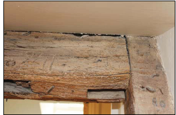
Assembly mark 'VI' to common-rafter, SF02, taken from the north-west
