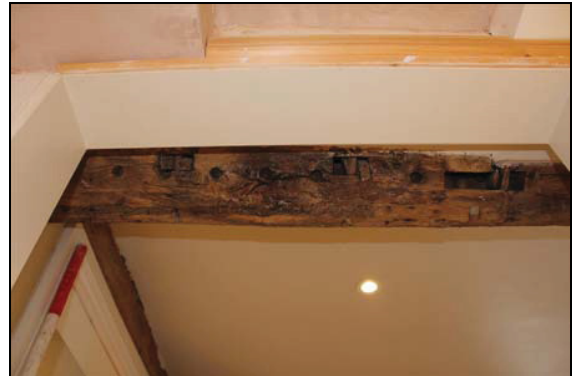
Eastern purlin with regular arrangement of pegs for common-rafters above and below, SF04, taken from the north-west
