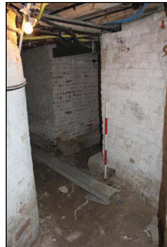
Ceiling to the basement formed of large chamfered central joist and chamfered common-joists with lamb tongue chamfer stops, BF01, taken from the west
