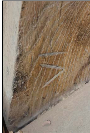
Assembly mark 'VI' to common-rafter, SF02, taken from the north-west
