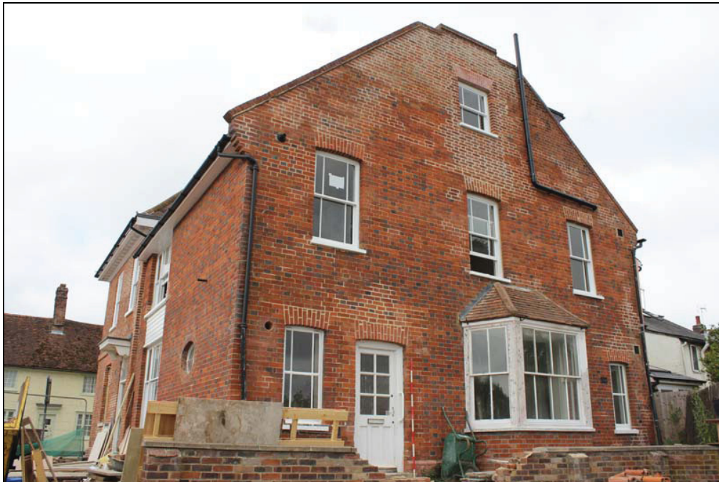
Plate 7 East elevation, taken from the south-east (DP78)
