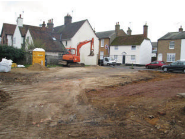
DP 1. The site. Looking south.
