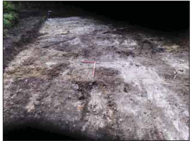
2 Area of new pool looking south
