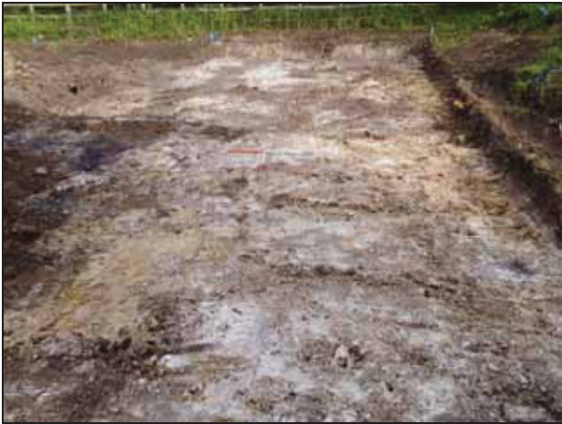
1 Area of new pool looking north
