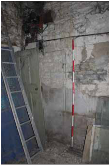
West wall of the barn showing blocked doorway indicated by a straight joint in the stonework, taken from the north-east
