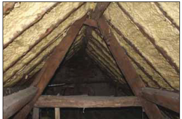
West end of the main range at roof level showing change in fabric reflecting the raising of the eaves (indicated), taken from the south-west
