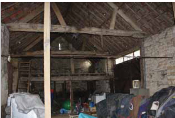
West wall of the barn showing blocked doorway indicated by a straight joint in the stonework, taken from the north-east
