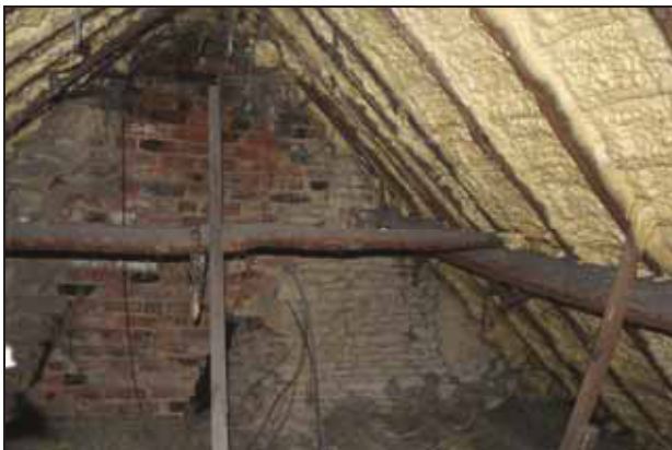
Detail in the roof space of the main range showing the through purlin and empty mortices for the original rafters (indicated), taken from the north-east
