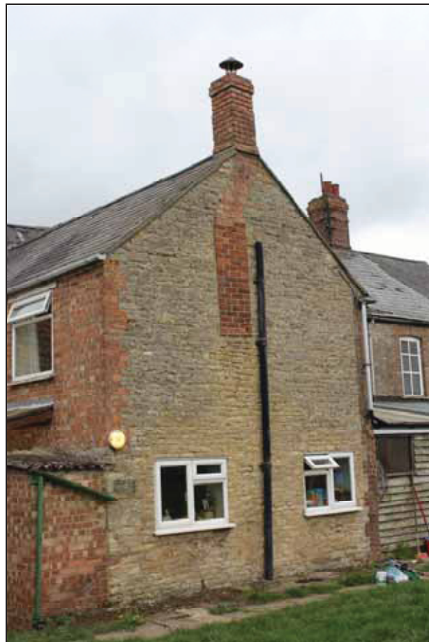
Plate 2 North elevation of the rear range, taken from the north-east (DP 04)
