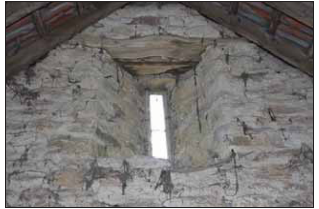
Detailed view of the high-set ventilation aperture in the east gable end of the barn, taken from the west
