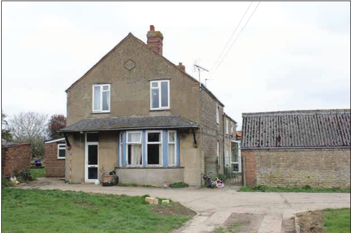
Plate 3 West gable end of west range, taken from the west (DP 1)
