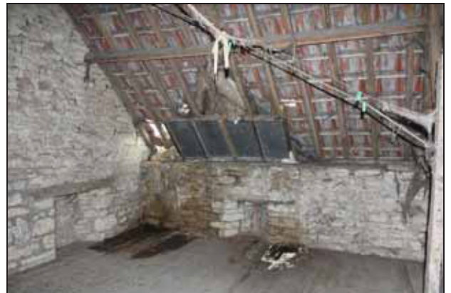
East end of the barn below the inserted floor showing bisected ventilation apertures, taken from the west
