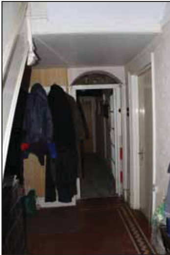
39 Entrance hall GF05 in the west range, taken from the west
