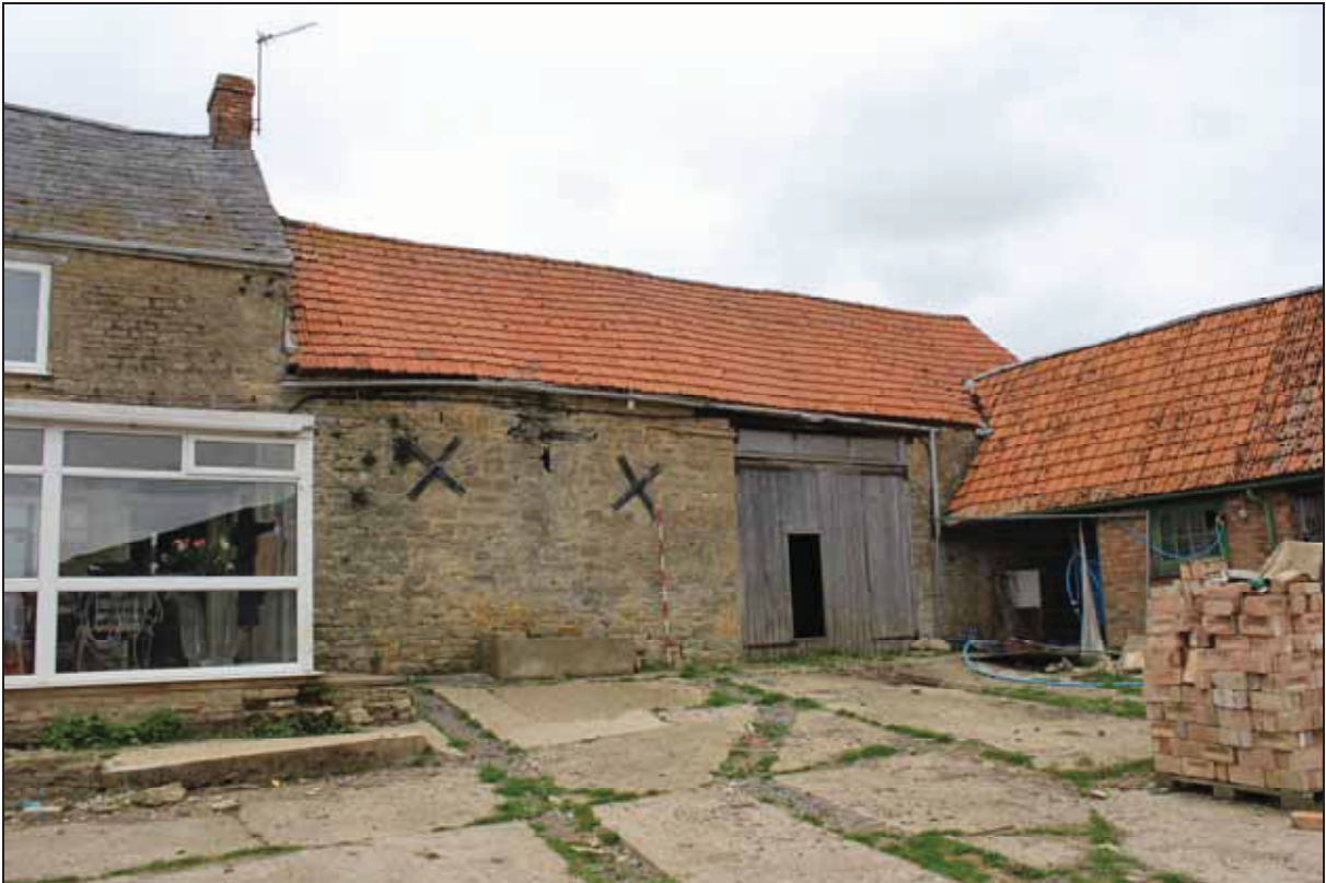
Plate 8 South elevation of the barn, taken from the south-west (DP 14)
