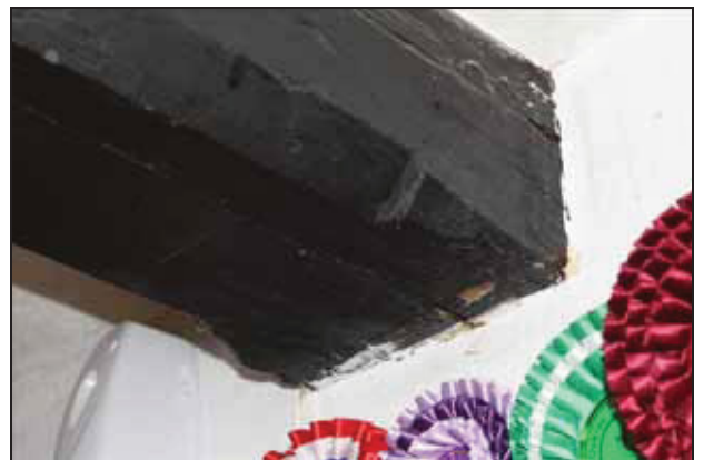
Detail showing a lambs tongue chamfer stop on the binding joist in Room GF01 (main range), taken from the north-west
