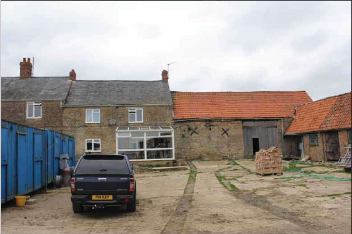
Plate 1 South elevation of the main range and barn, taken from the south (DP 01)
