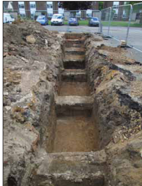
4. General shot of modern footings Trench 2, facing east.
