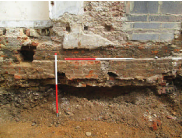
DP 3. Exposed foundations of No. 114-116. Looking north-east.
