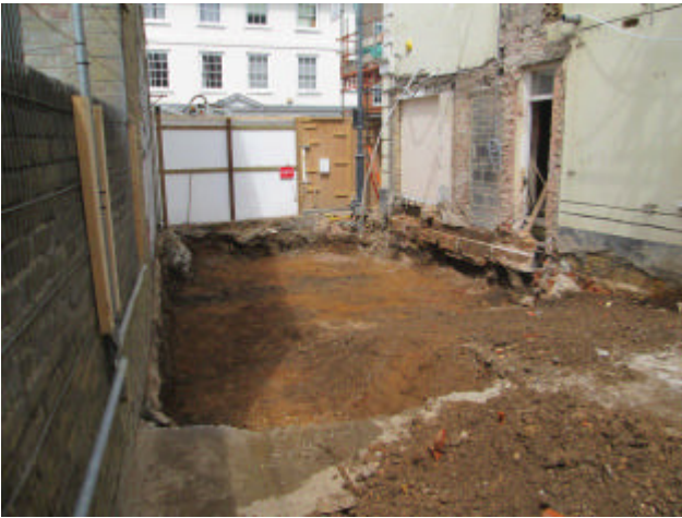
DP 1. The area of excavation. Looking north-north-west.
