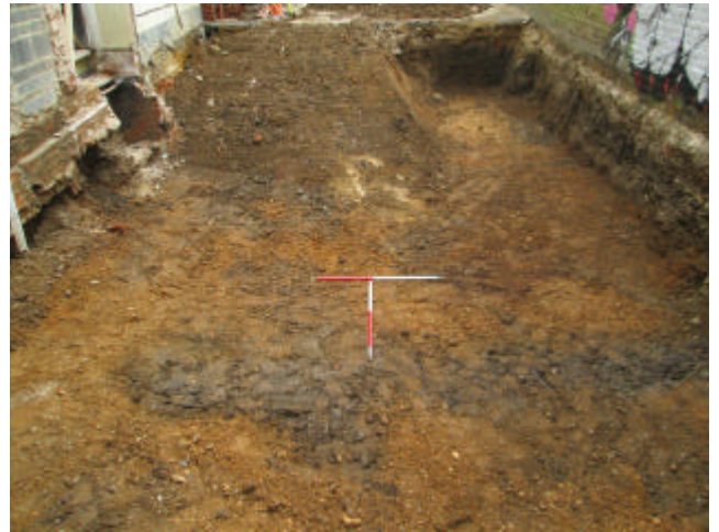
DP 2. The area of excavation. Looking south-east.
