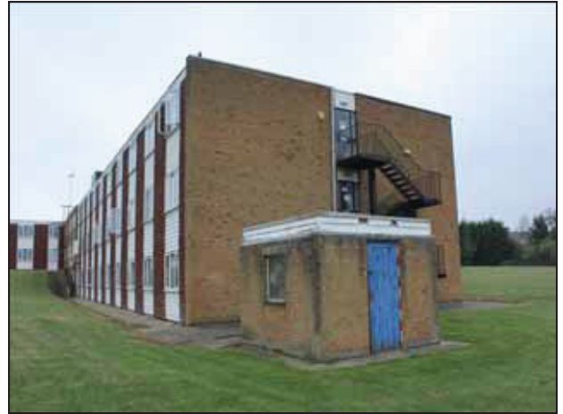
14 Rear range and sub-station building, taken from the north-west.
