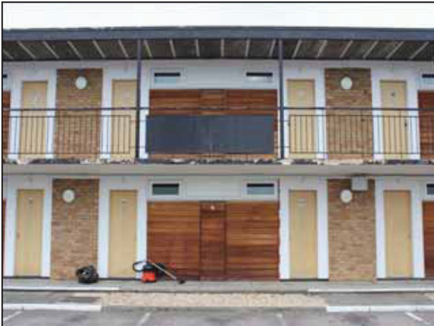
5 Southern wing of the main frontage, taken from the east.
