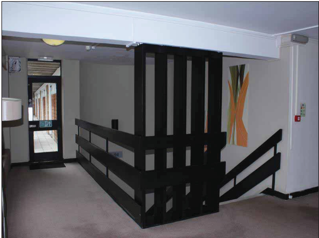
Plate 6 FF01, first floor lobby, showing the 1970s original staircase, taken from the north (DP 36)
