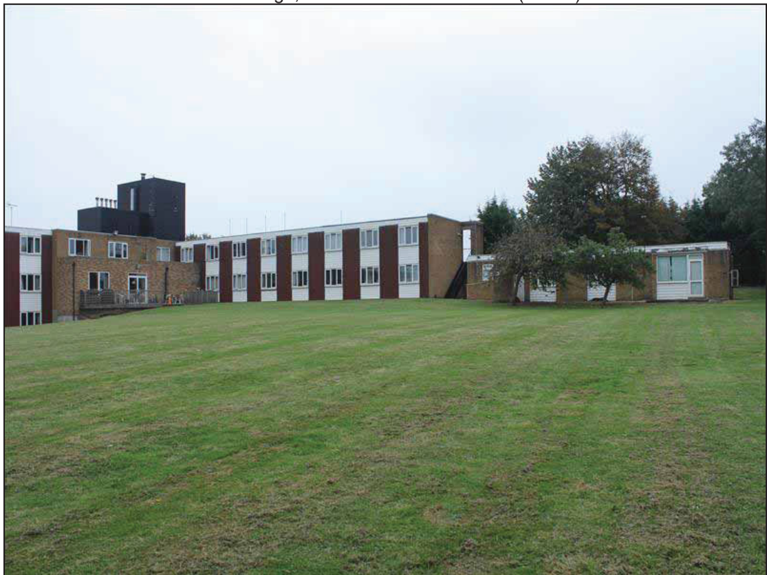
Plate 4 Rear south facing single story extension and the manager's bungalow at the southern end of the building, taken from the south-west (DP 8)
