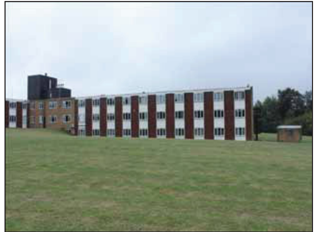
16 General shot of the rear range of the building, taken from the north.
