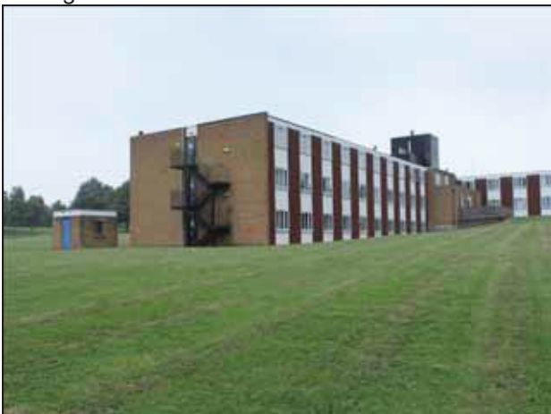
11 Western end of the rear range and sub-station building, taken from the west.
