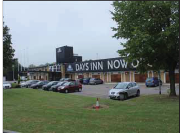
2 General shot of the motel building, taken from the north-east.
