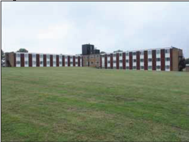
15 Rear range and northern wing of the main frontage, taken from the north.
