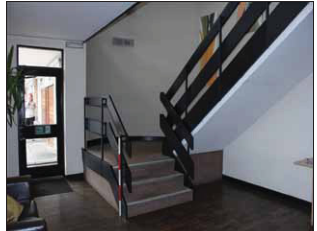
20 Shot of the stair case in the main reception area (GF01).
