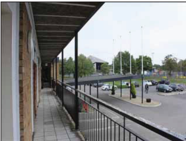
39 Corridor providing access to guest rooms on the first floor southern wing of the main frontage, taken from the south-west.
