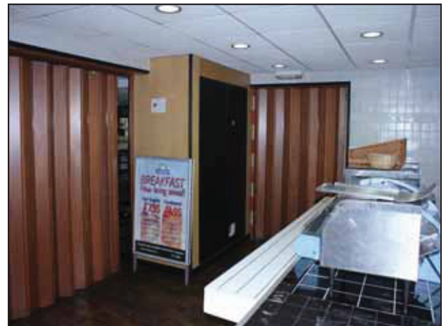
24 Shot of servery and kitchen area, taken from the south.
