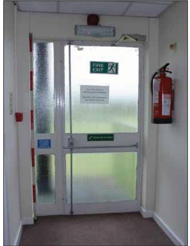
38 Fire exit at the north-western end of the first floor corridor.
