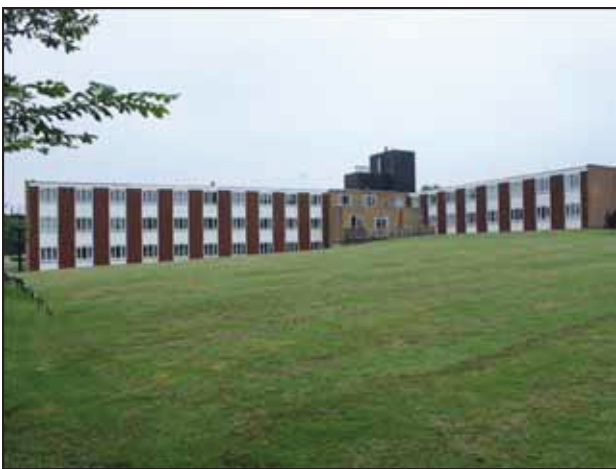
9 General shot of the rear of the building, showing the rear range and the southern wing of the main frontage. Taken from the south-west.
