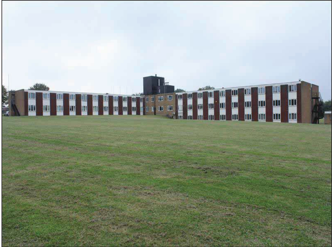
Plate 3 General shot of the rear central block and rear of the northern wing of the main frontage, taken from the north-west (DP 15).
