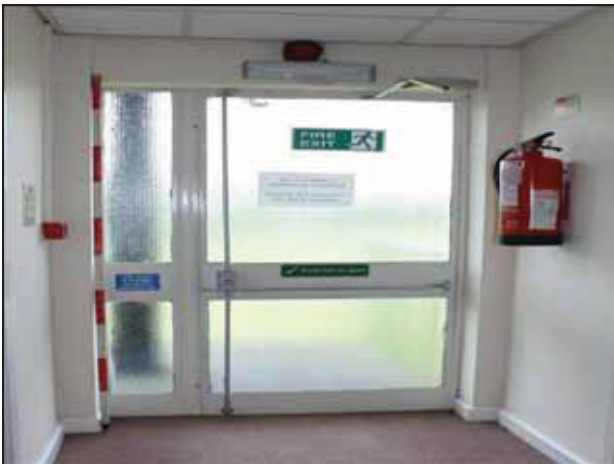
27 Fire exit, situated at the end of the ground floor corridor, taken from the east.
