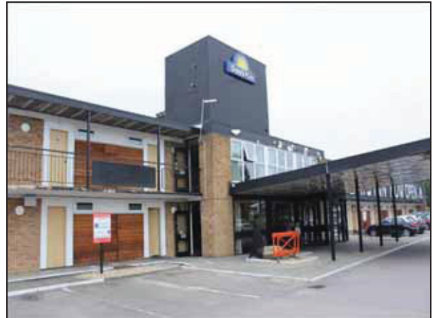
6 General shot of the main frontage, taken from the south-east.
