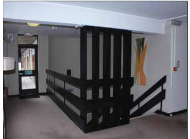
36 FF01, showing 1970s style staircase, taken from the north-east.
