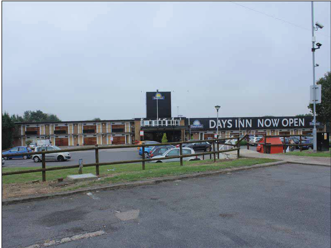
Plate 1 Main frontage of the building, taken from the east (DP 3)
