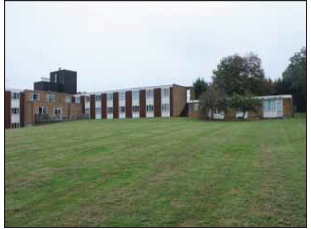
8 General shot of the rear of the building, showing the southern wing and the manager's bungalow, taken from the west.
