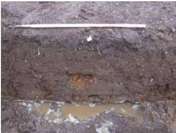
DP3: Sample Section 1 (including modern Drain F1006), looking S
