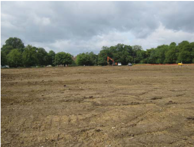
DP 9. The area of grass pitches. Looking west-north-west.
