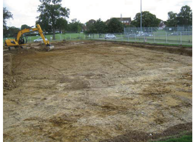
DP 8. Reducing the ground within the synthetic pitch area. Looking east.
