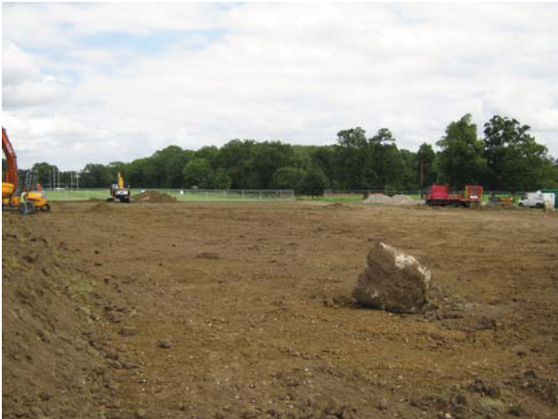
DP 3. Western part of the synthetic pitch area. Looking east.
