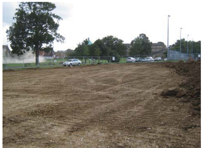
DP 6. Southern part of the synthetic pitch area. Looking south-south-west.
