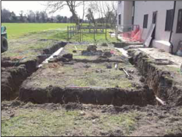
1 General shot of site looking south.
