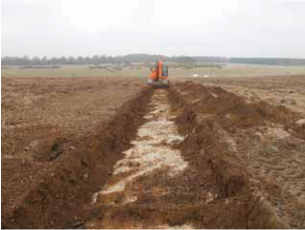
1 Excavating Trench 2, Looking northwest.
