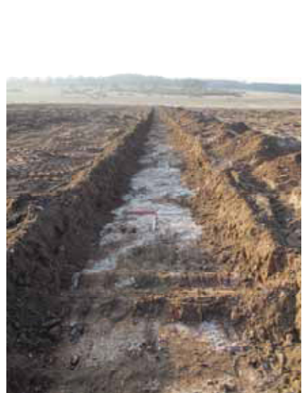
6 Trench 2 post exc, looking northwest.
