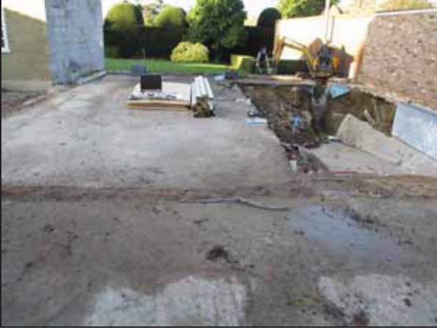
1 General shot showing concrete being broken up
