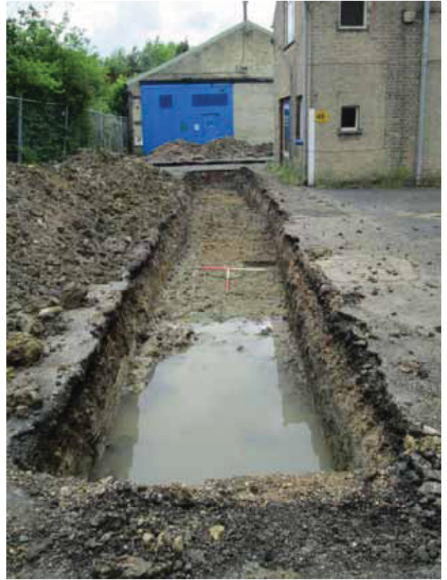
8 Post excavation shot of Trench 3
