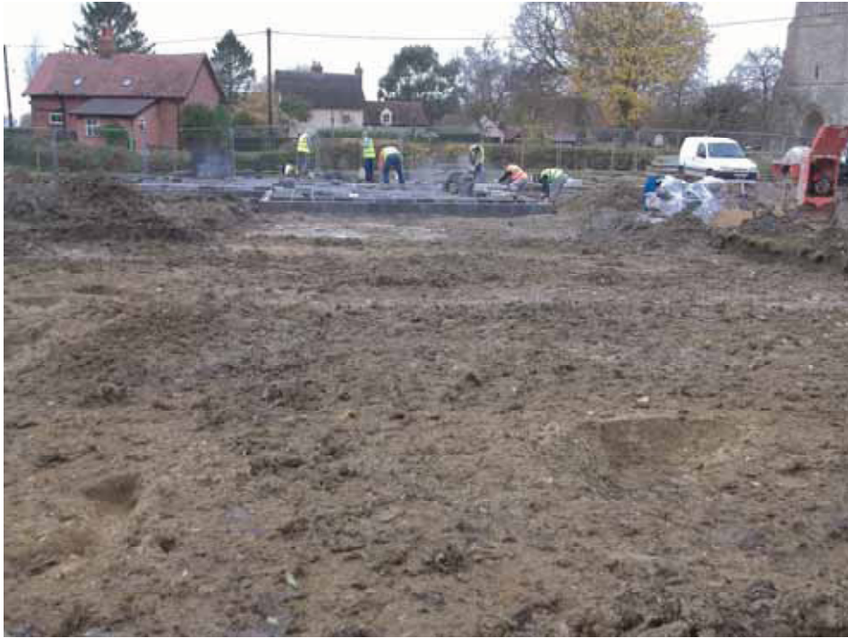
Plate 1: Site shot (post-excitation), looking NW
