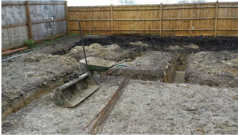
DP 1. Foundation trenches. Looking north.
