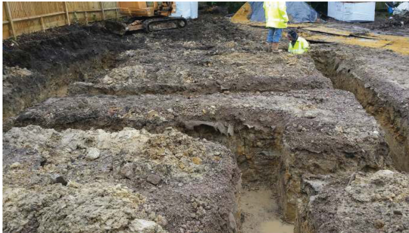
DP 2. Foundation trenches. Looking east-south-east.
