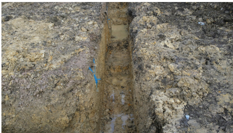
DP 3. North-east foundation trench. Looking south-south-west.
