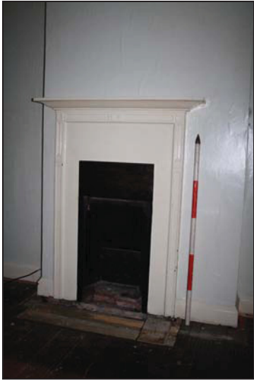
DP 19 Fireplace in Room FF02, taken from the west
