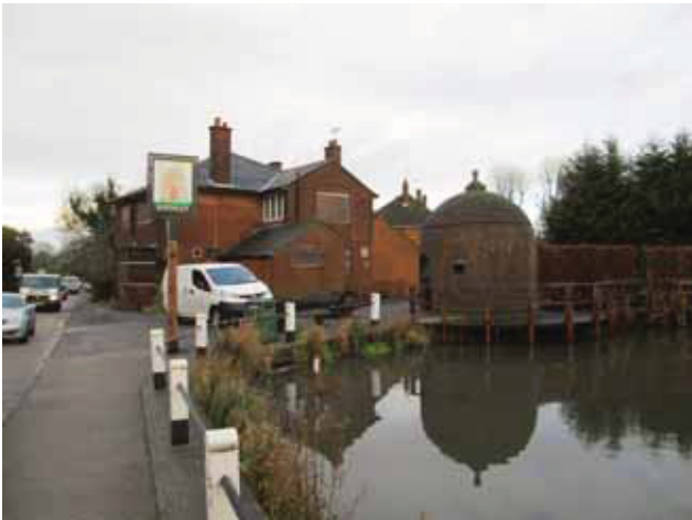
DP 1. Queen Adelaide PH, Shenley, Hertfordshire. Looking north-west.
