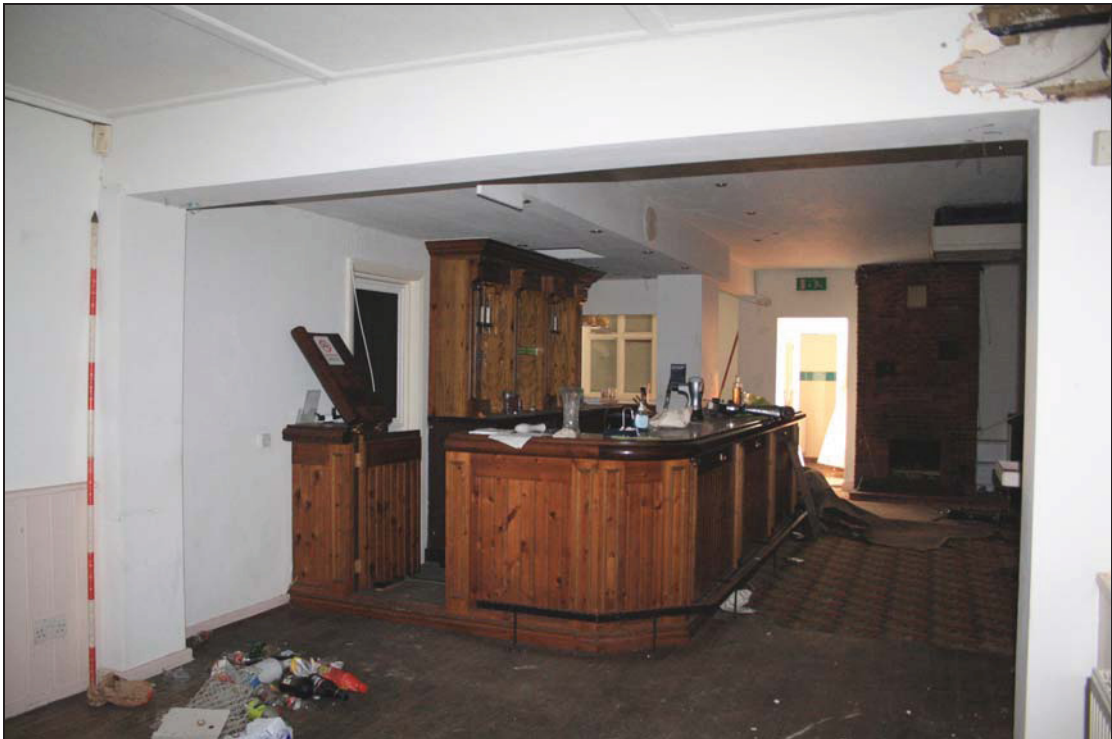
Plate 2 Main public bar area (GF01), taken from the west (DP 07)
