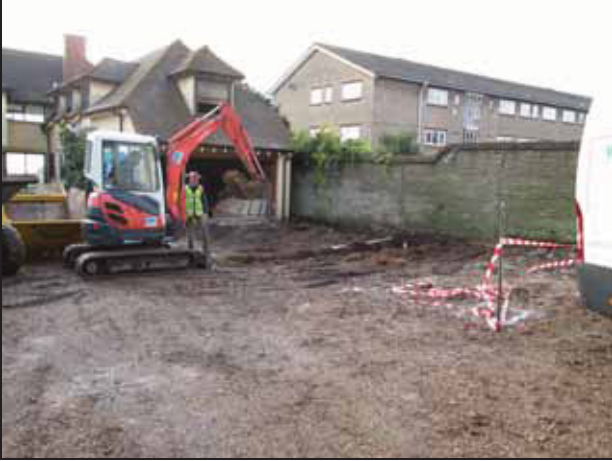
1 General shot of site before excavation
