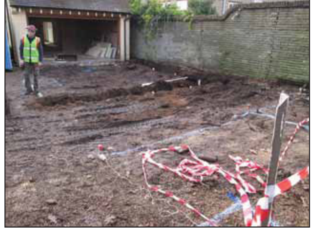
2 General site shot after footings excavated
