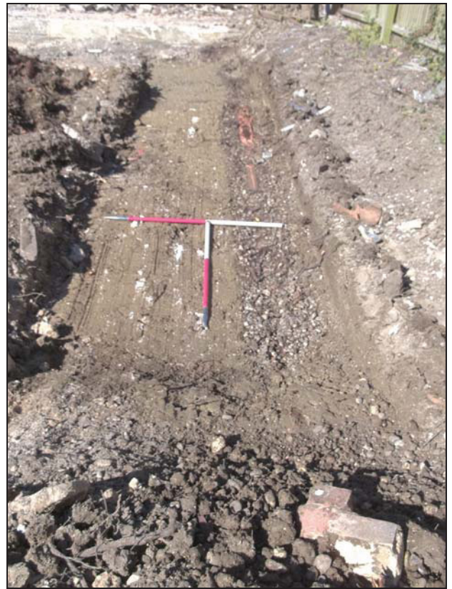
4 View of trench 2 looking south-west
