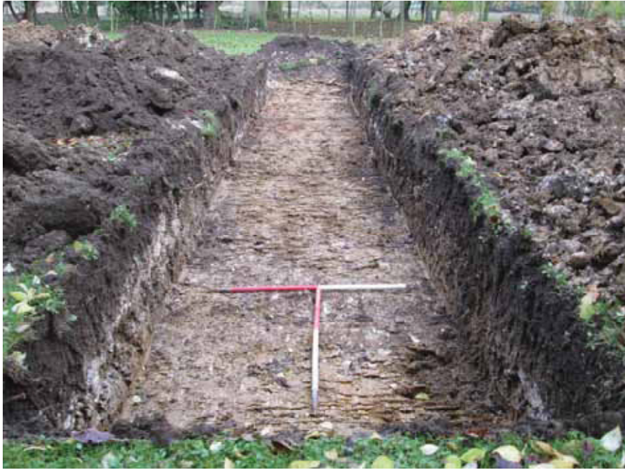
DP 5: Trial Trench 2 (post-excitation)
