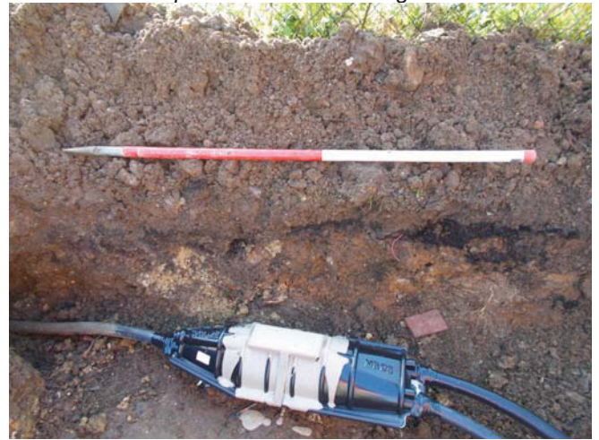
16 Sample Section 7. Looking south.
