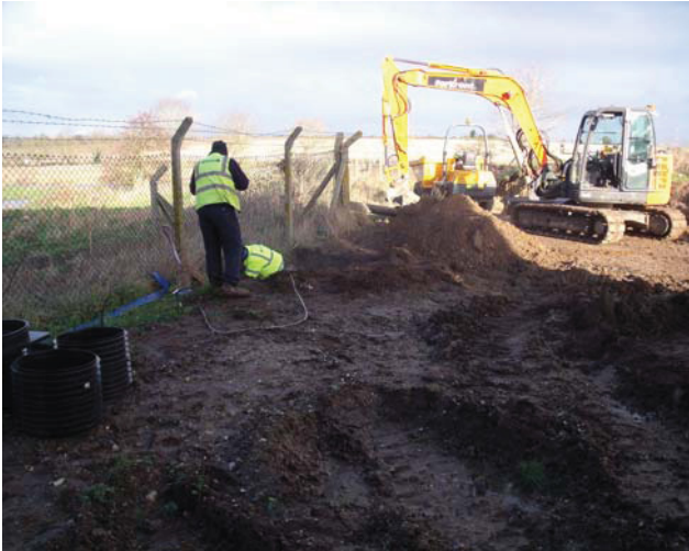
Excavating trench for septic tank. Looking north.
