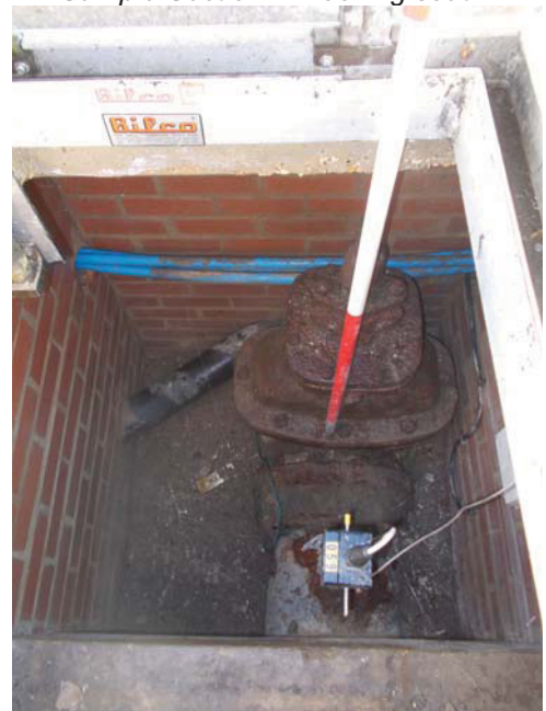
18 View down manhole adjacent to northern building.
