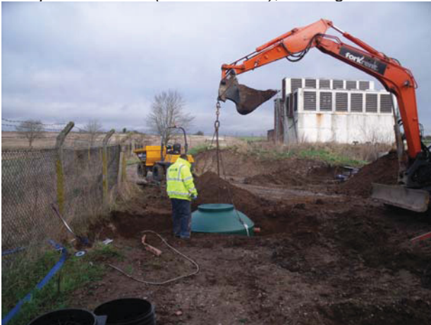
Placing septic tank. Looking north.
