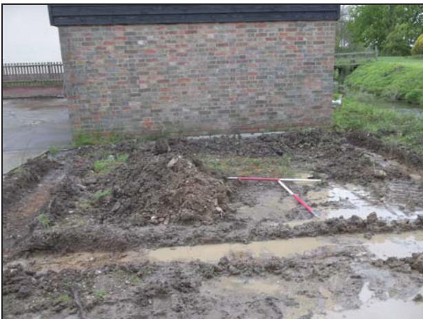
5 General view of Area 1 looking north-west
