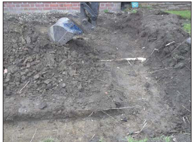
6 General view of Area 2 looking south-west
