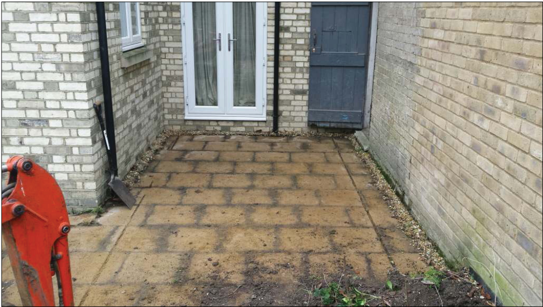
DP 1. Area of groundworks prior to excavation. View south-west
