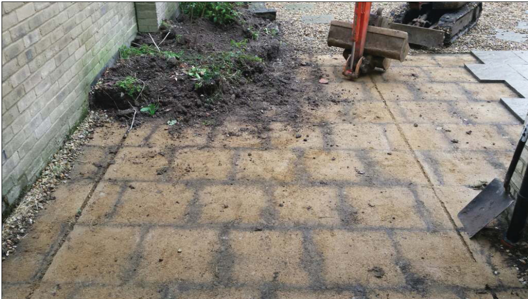
DP 2. Area of groundworks prior to excavation. View north-east
