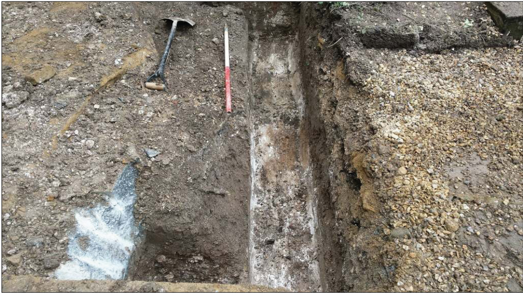
DP 5. Foundation Trench. View north-west
