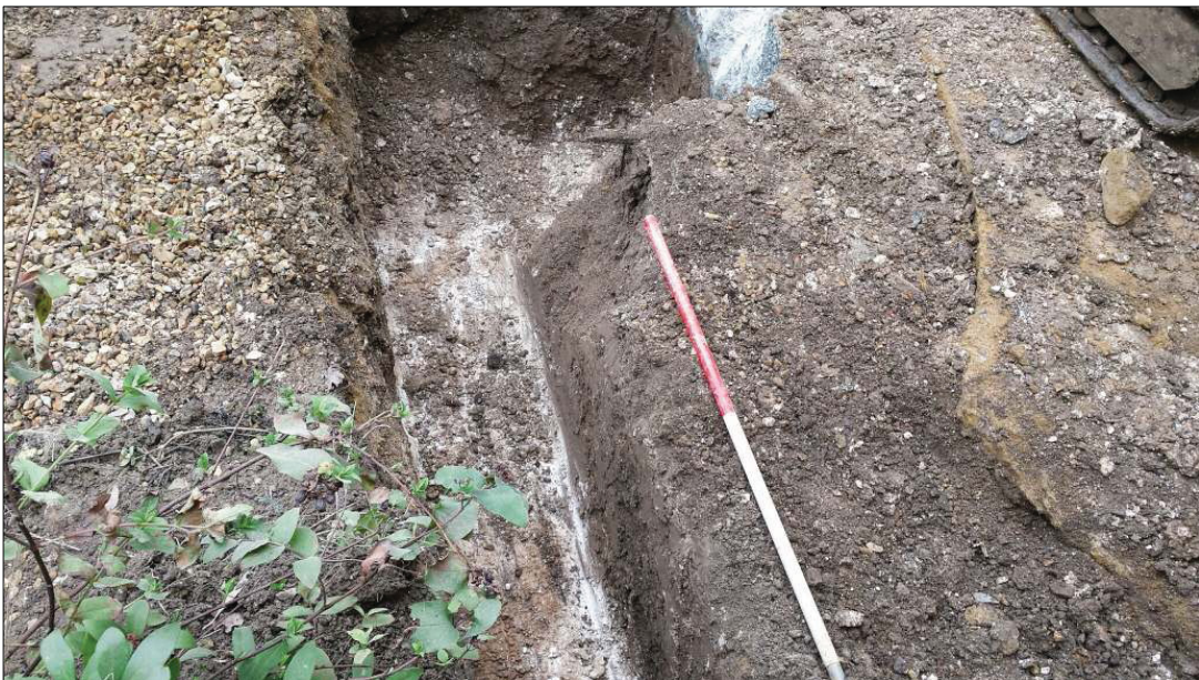
DP 6. Foundation Trench. View south-east
