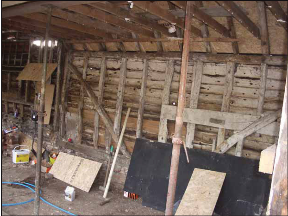
6.16 West wall of the north unit showing weatherboarding to the rear. The sole-plate is visible as well a small section of the brickwork of the dwarf wall.
