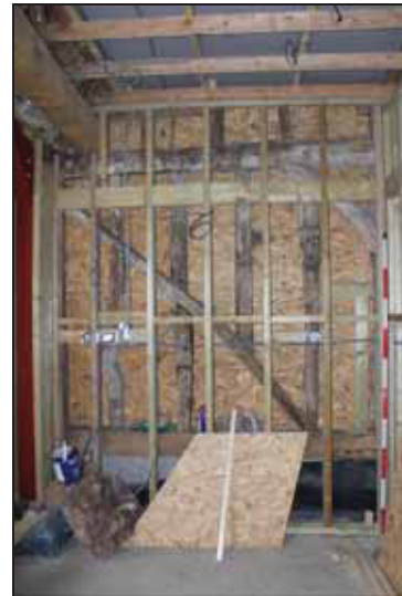
DP 22 View of the south wall showing primary-braced studwork (Area 1), taken from the north
