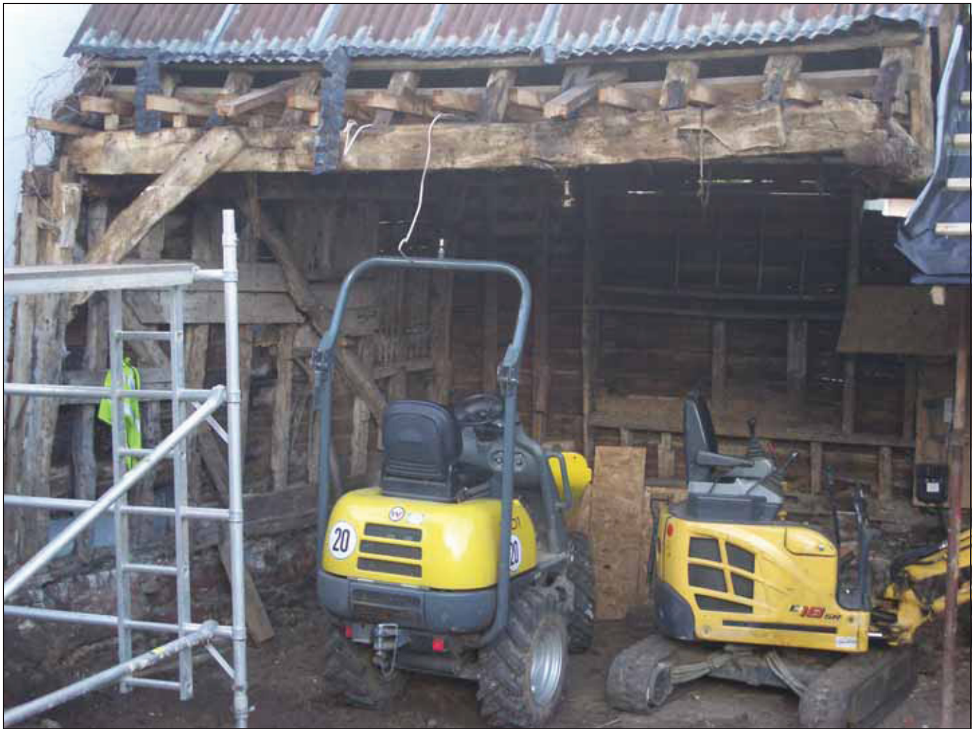
6.9 View into the south unit during planned works.
