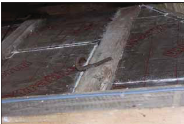
DP 11 Detail of the north wall (Area 2) showing a hook attached to a stud above tie-beam level, taken from the south
