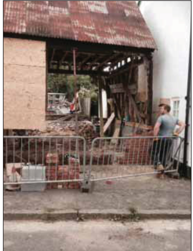
6.4 Working shot during the planned works. This shows the dwarf wall and sole-plate on the west removed as well as the pent-roofed unit on the east.
