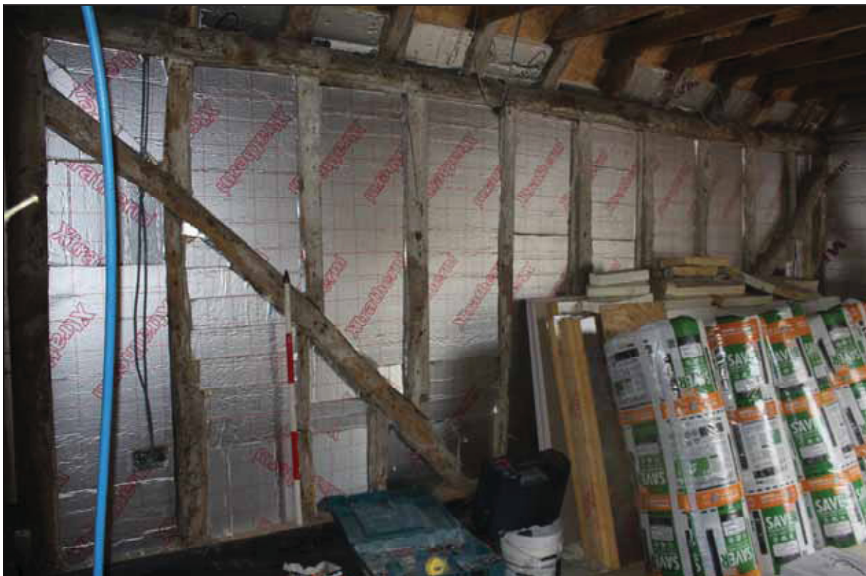
Plate 4 West wall of Area 2, taken from the south-east (DP 8)
