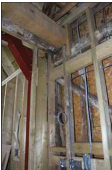
DP 23 Detail of the south-east corner post showing binding joist offset from the position of the bay post, taken from the north-west
