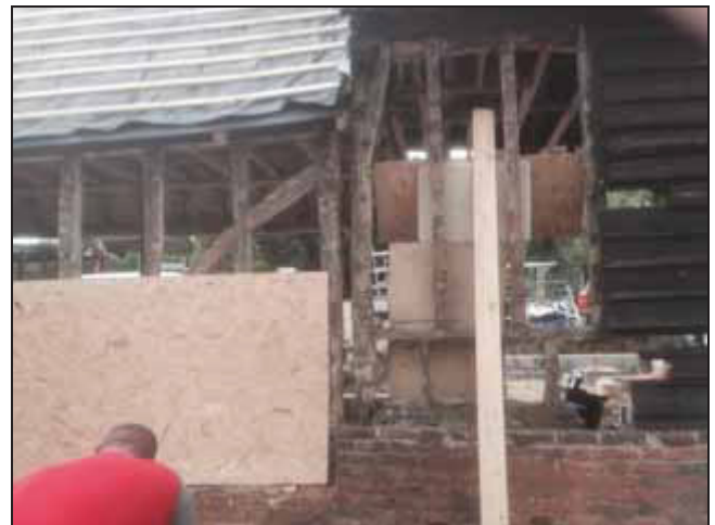
6.4 Working shot during the planned works. This shows the dwarf wall and sole-plate on the west removed as well as the pent-roofed unit on the east.
