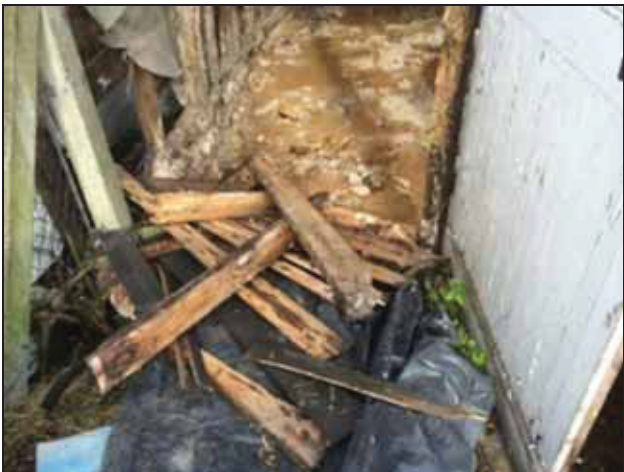
6.12 Area of the east pent-roofed extension with removed studs
