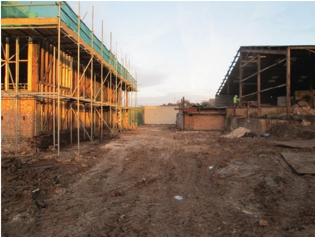
DP 3. Yard to the north-east of north barn (Units 3 & 4). Looking north-west.
