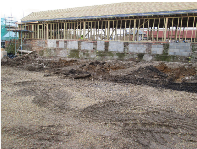
DP 5. Groundworks for extension to east barn (Unit 5). Looking west.
