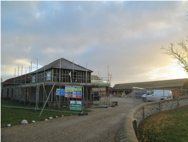
DP 1. Lordship Farm, Dane End. Looking east.
