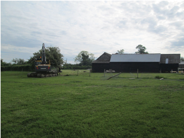
DP 1. The site. Looking east-north-east.
