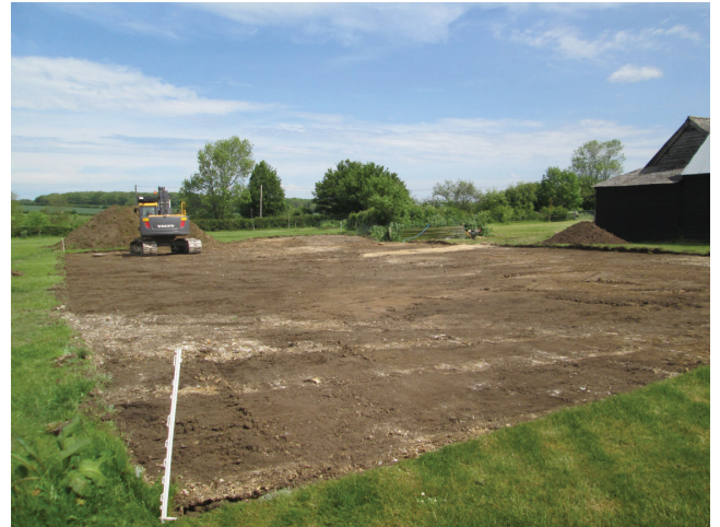
DP 2. Initial removal of topsoil. Looking north.
