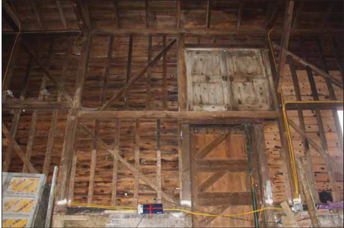
Plate 3 West side of Bay 4 showing the conventional door in the lower register and pitching door in the upper (DP 04)
