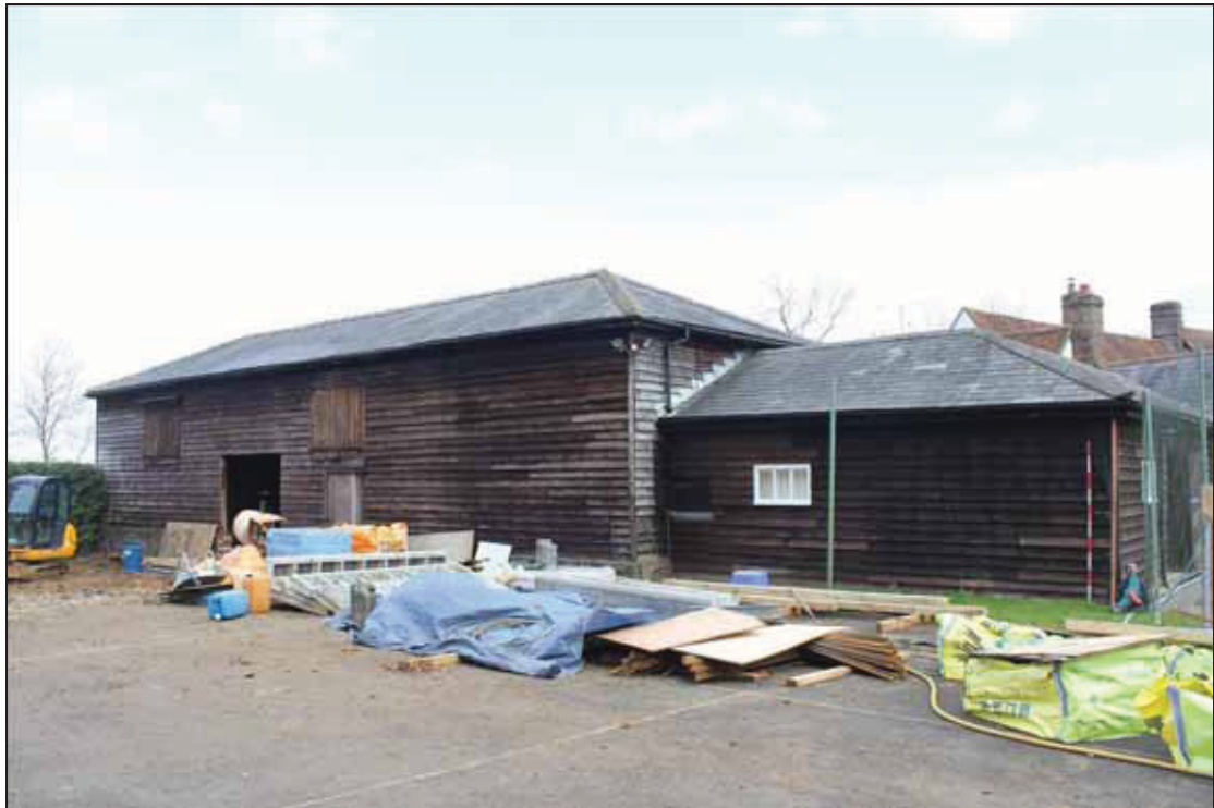
Plate 1 East elevation of the Barn, taken from the south-west (DP 23)
