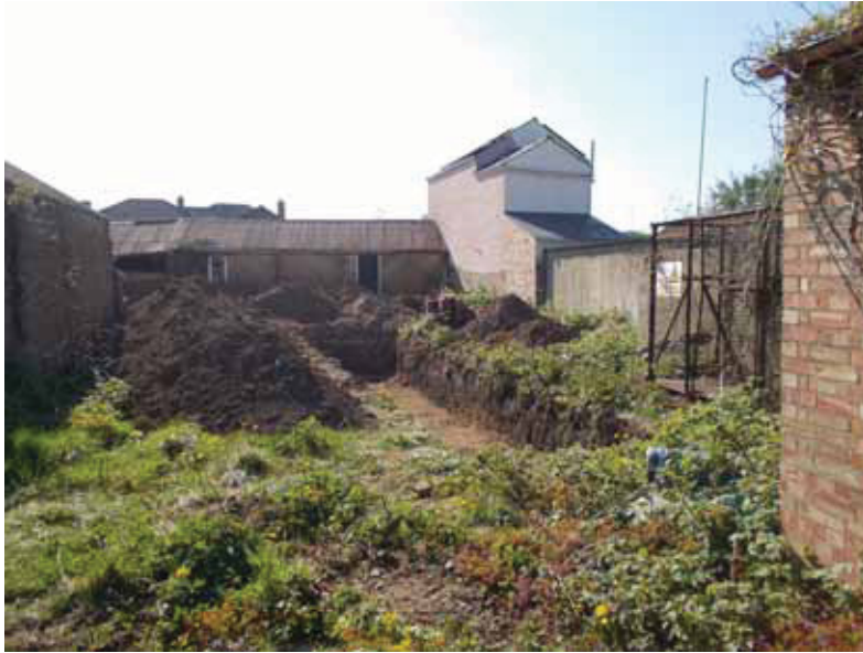
DP1: General site shot, SE corner looking NW
