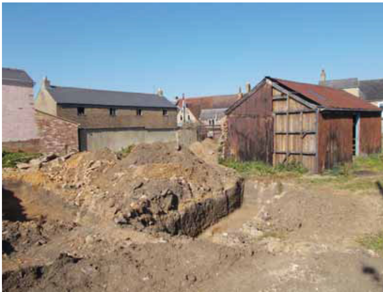
DP2: General site shot, SW corner looking NE
