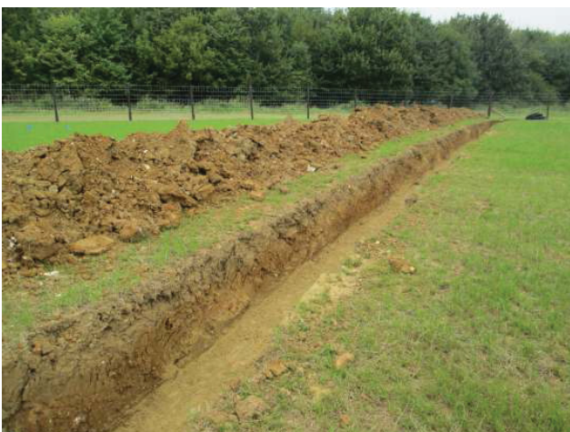
DP 17. Trench in north part of solar farm. Looking north-east.
