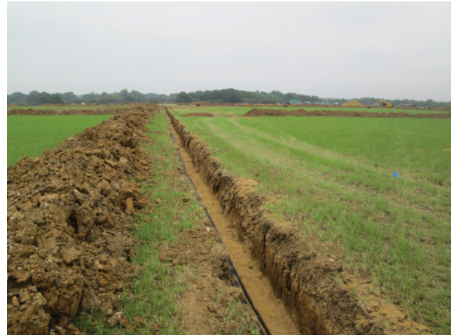
DP 20. Trench in west part of solar farm. Looking south-east.
