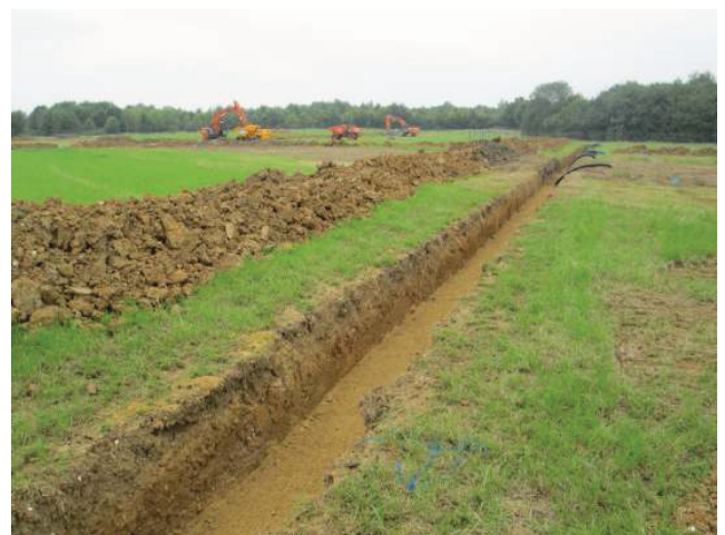
DP 18. Trench in north part of solar farm. Looking north-east.
