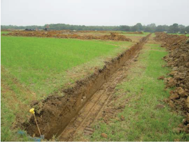
DP 13. Trenches in central part of solar farm. Looking north-east.
