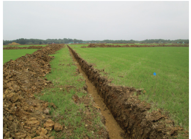
DP 22. Trench in west part of solar farm. Looking north.
