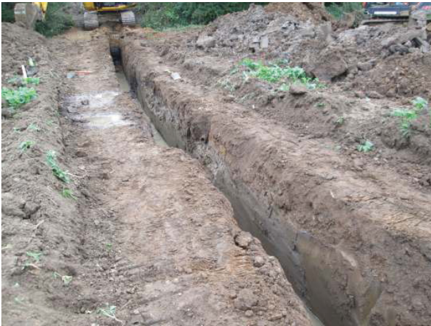
DP 3. South section of power grid connection trench. Looking south-west.
