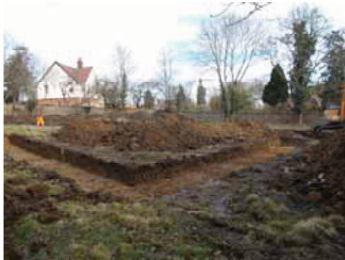
DP13: General site shot, looking N
