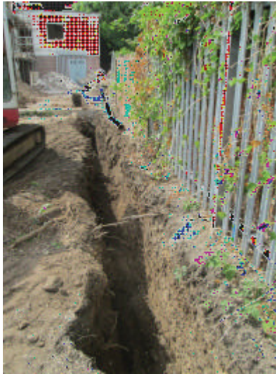
DP 3. Service trench. Looking west.
