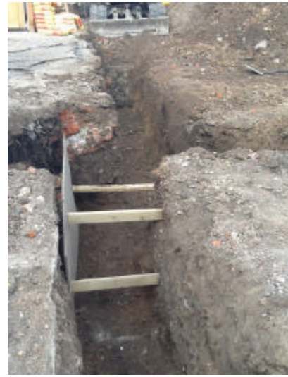
DP 8. South foundation trench. Looking west.
