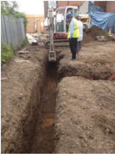
DP 7. North foundation trench under excavation. Looking east.
