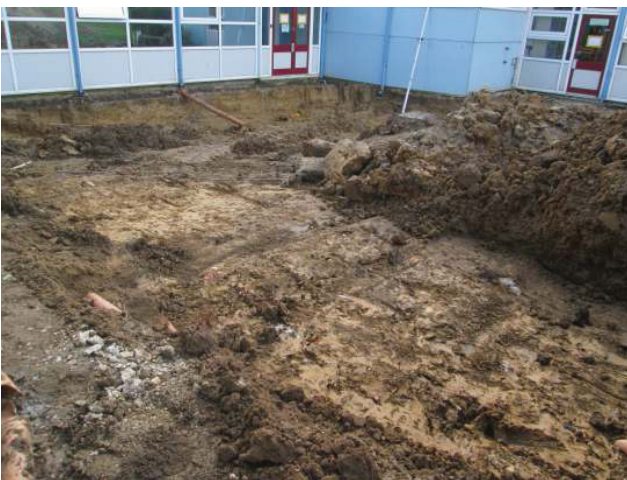
DP 5. North part of the site. Looking south-east.
