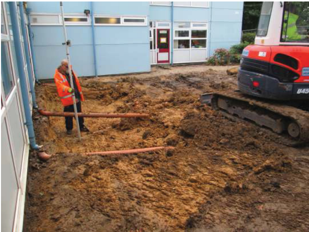
DP 3. East part of the site during further excavation. Looking south-south-west.
