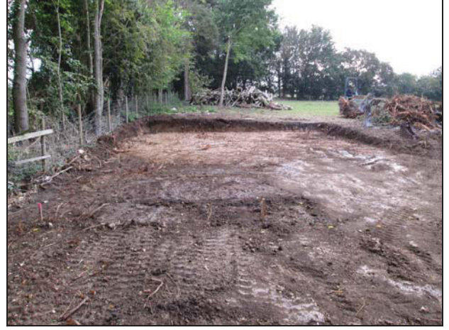
2 View of excavation area looking north-east
