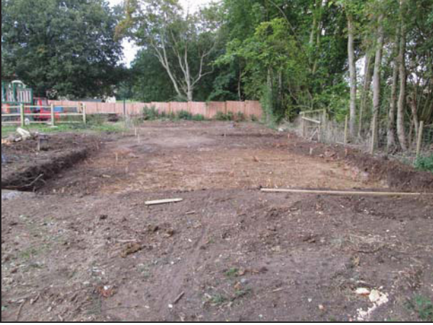
1 View of excavation area looking south-west
