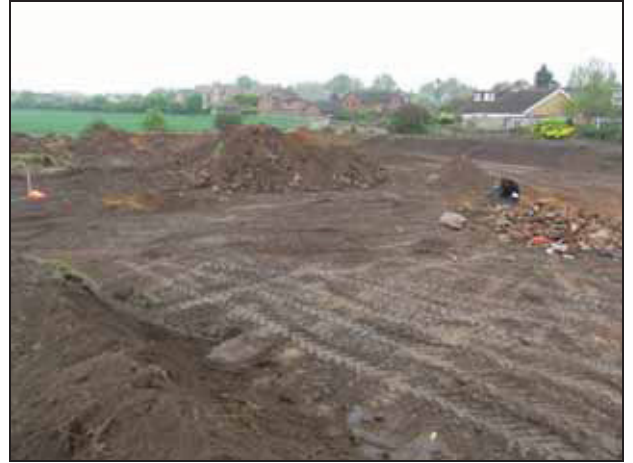
2 General view of site before commencement of works
