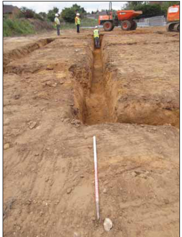
4 General shot of footings
