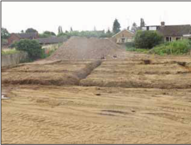
5 General shot of footings
