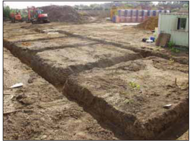
6 General shot of footings
