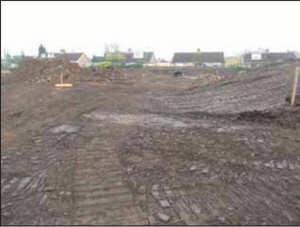
1 General view of site before commencement of works
