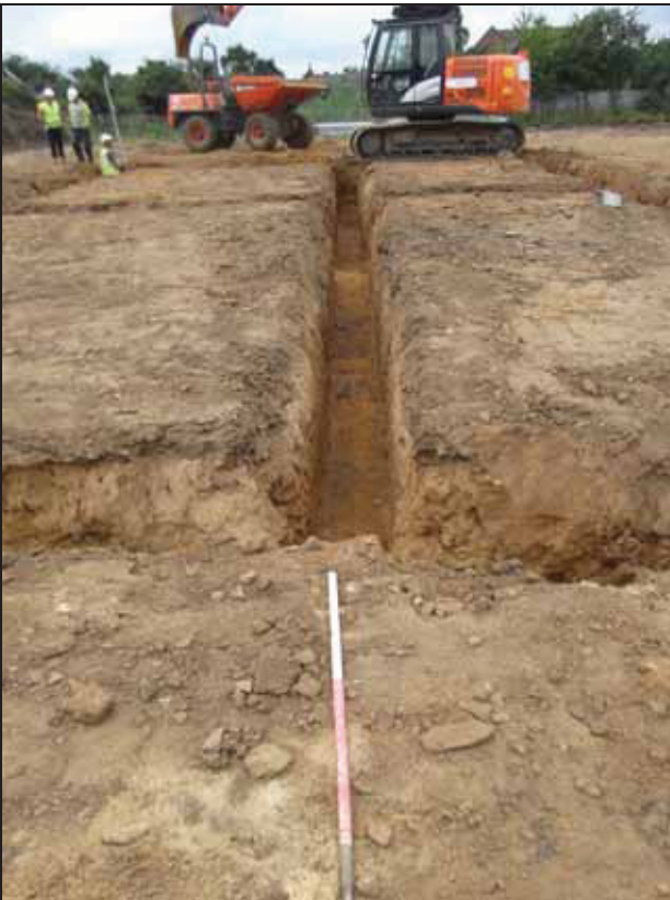
3 General shot of footings
