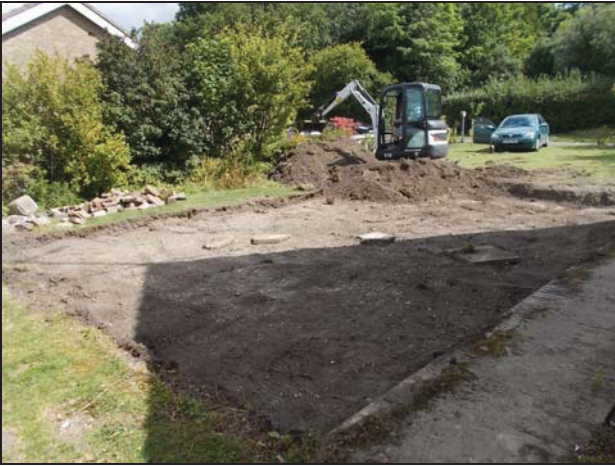
5 Pre-excitation view of site looking east
