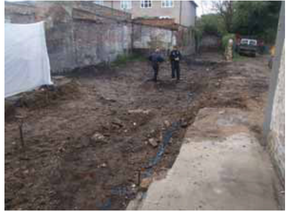
DP 2: Site shot (pre-excitation), looking S
