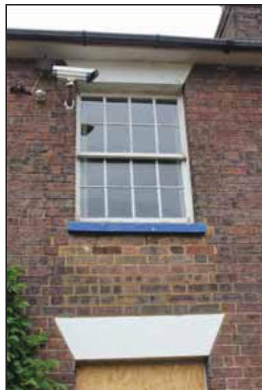
Detail of the west elevation of No. 32 showing disturbed brickwork below the northern first floor window, taken from the west
