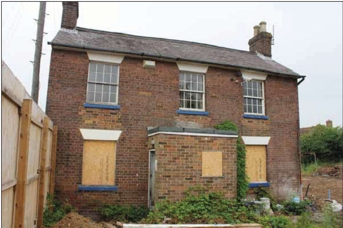
Plate 2 West elevation of No. 32, taken from the west (DP 9)
