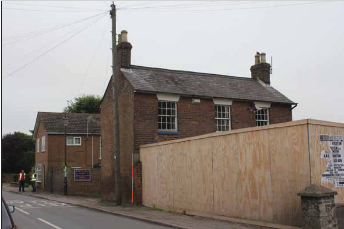
Plate 1 View of No. 32 with Nos. 26-28 to the rear both with their short elevations fronting the street, taken from the west (DP 02)
