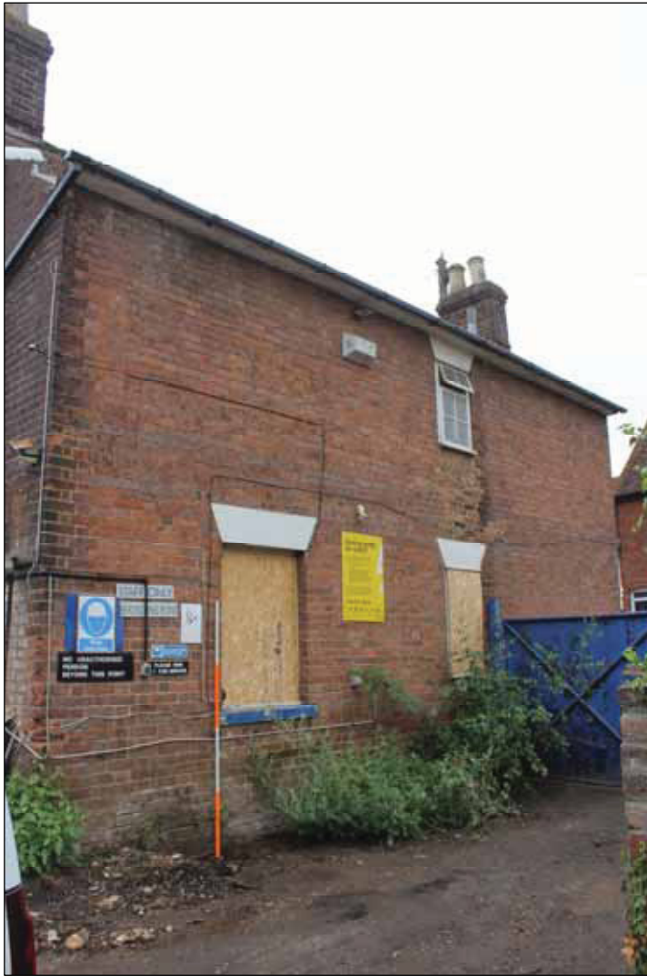
Plate 3 East elevation of No. 32, taken from the south-east (DP 14)
