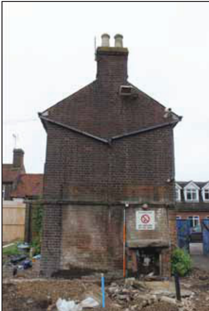
DP 15 South elevation of No. 32, taken from the south
