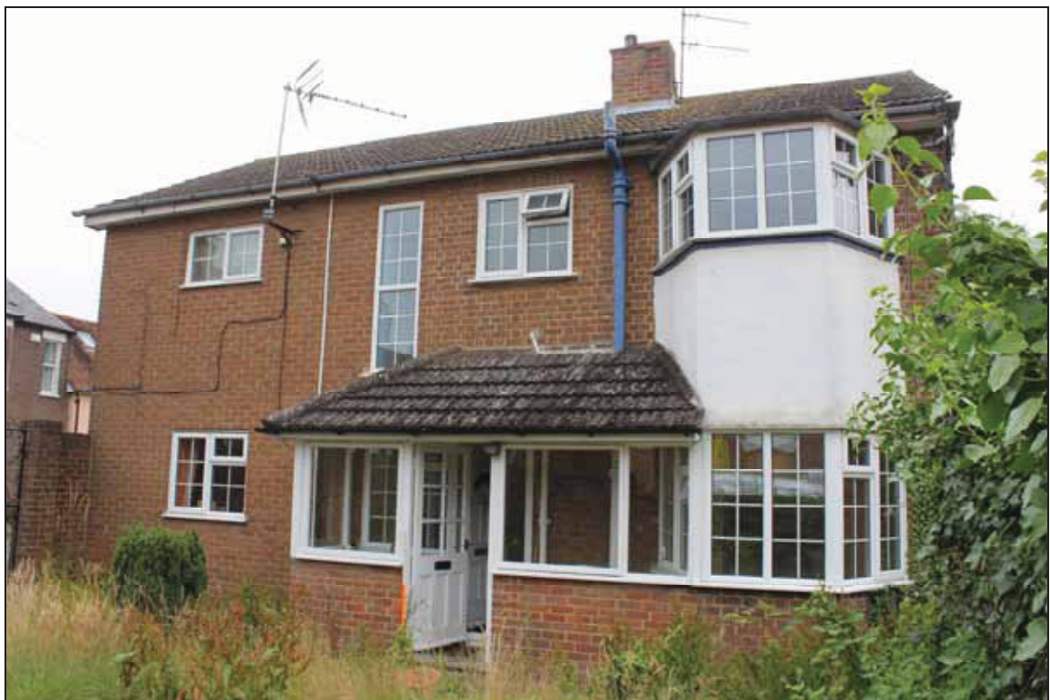
Plate 9 West elevation of No. 26-28, taken from the west (DP 17)
