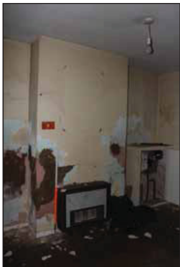
DP 23 Projecting chimney breast on the north side of Room GF02 (No. 32), taken from the south-west
