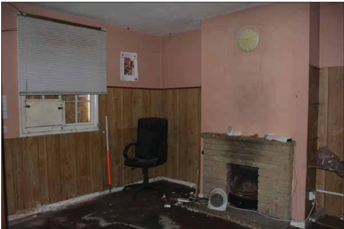
Plate 4 Chimney breast and replacement sash window in Room GF05 (No. 32), taken from the north-west (DP 27)
