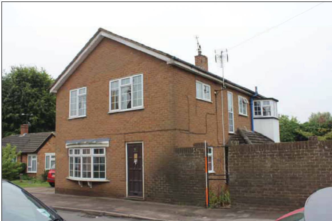
Plate 7 North and west elevations of Nos. 26-28, taken from the north (DP 5)
