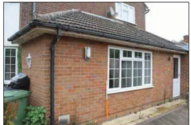
DP 18 Modern single-storey extension at the south end of Nos. 26-28, taken from the south-west
