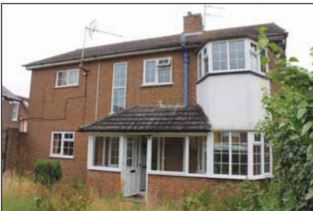
DP 17 West elevation of No. 26-28, taken from the west
