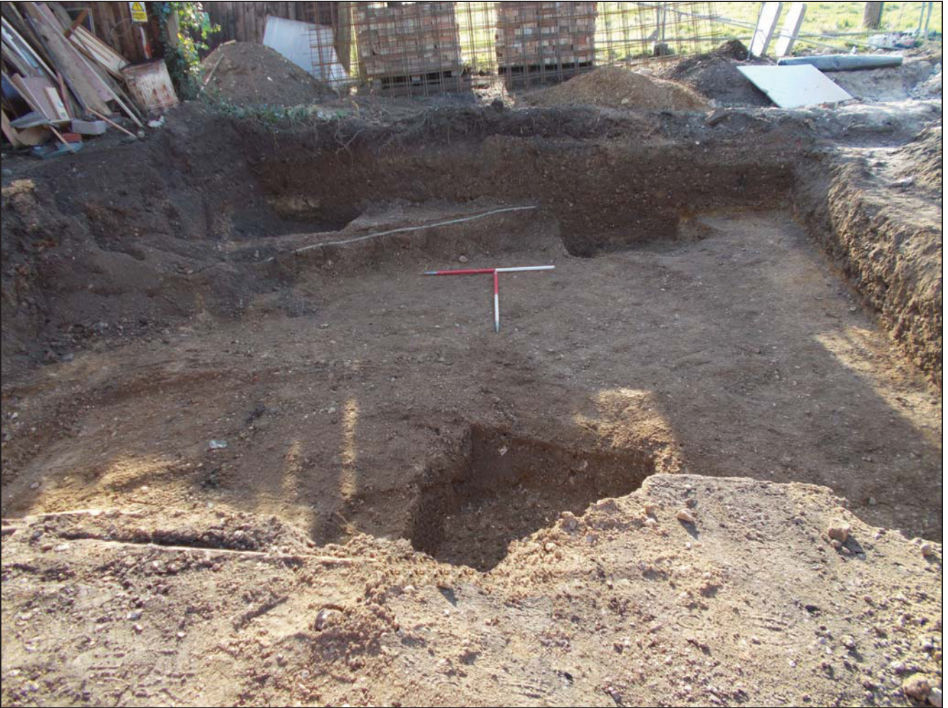
1 Post-excitation view of site looking south-west.
