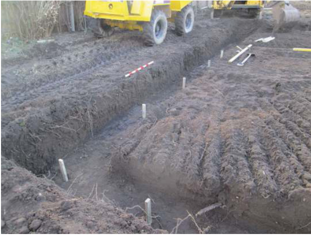
DP 7. South foundation trench. Looking south-west.
