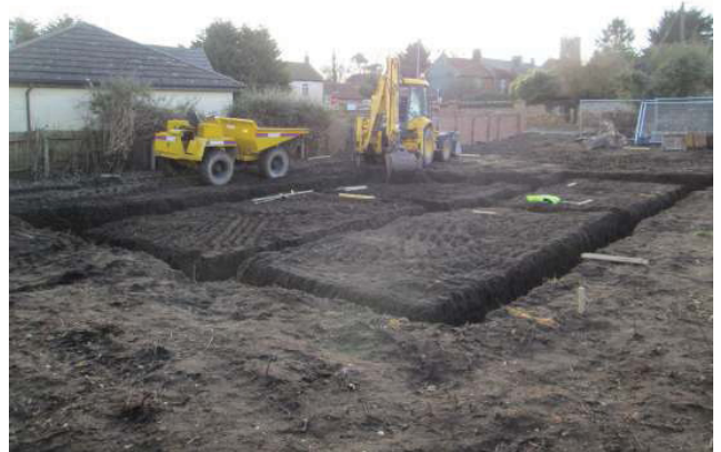
DP 2. Excavated foundation trenches for new house. Looking south-west.
