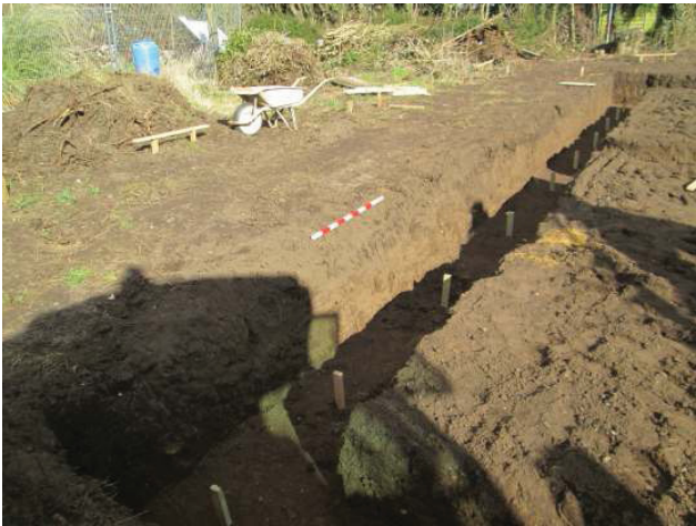
DP 3. North foundation trench. Looking north-east.
