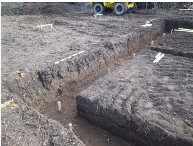
DP 5. East foundation trench. Looking south-east.
