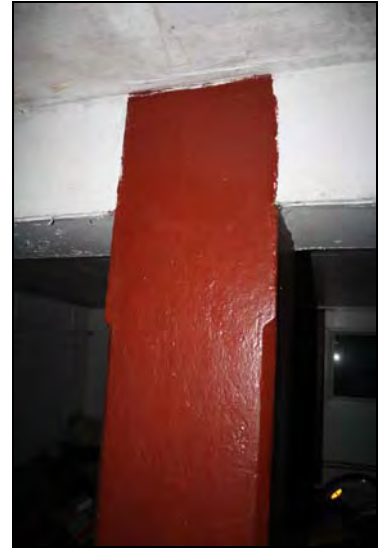
DP 98 Detail of an original pre-cast concrete column in Range 9 (GF21) showing chamfered and stopped corners, taken from the south
