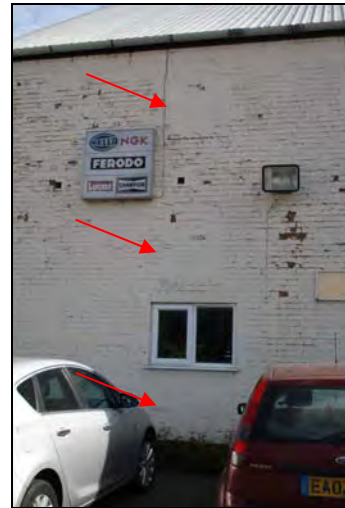
DP 4 Detail of the south elevation (Range 1) showing small blocked apertures marking three original floor levels, taken from the south
