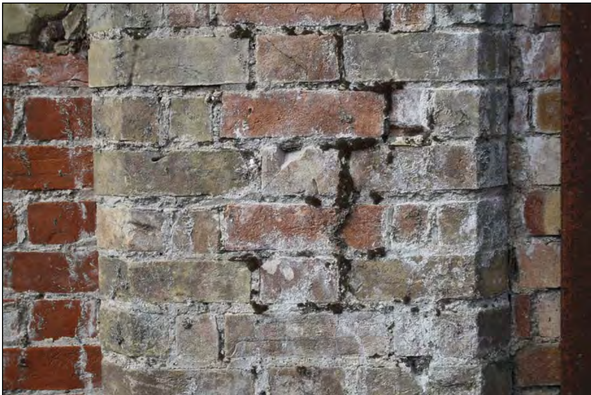
Plate 2 Detail of the north elevation (Range 1) showing original brick pilaster with chamfered gault brick corners, taken from the north (DP 59)
