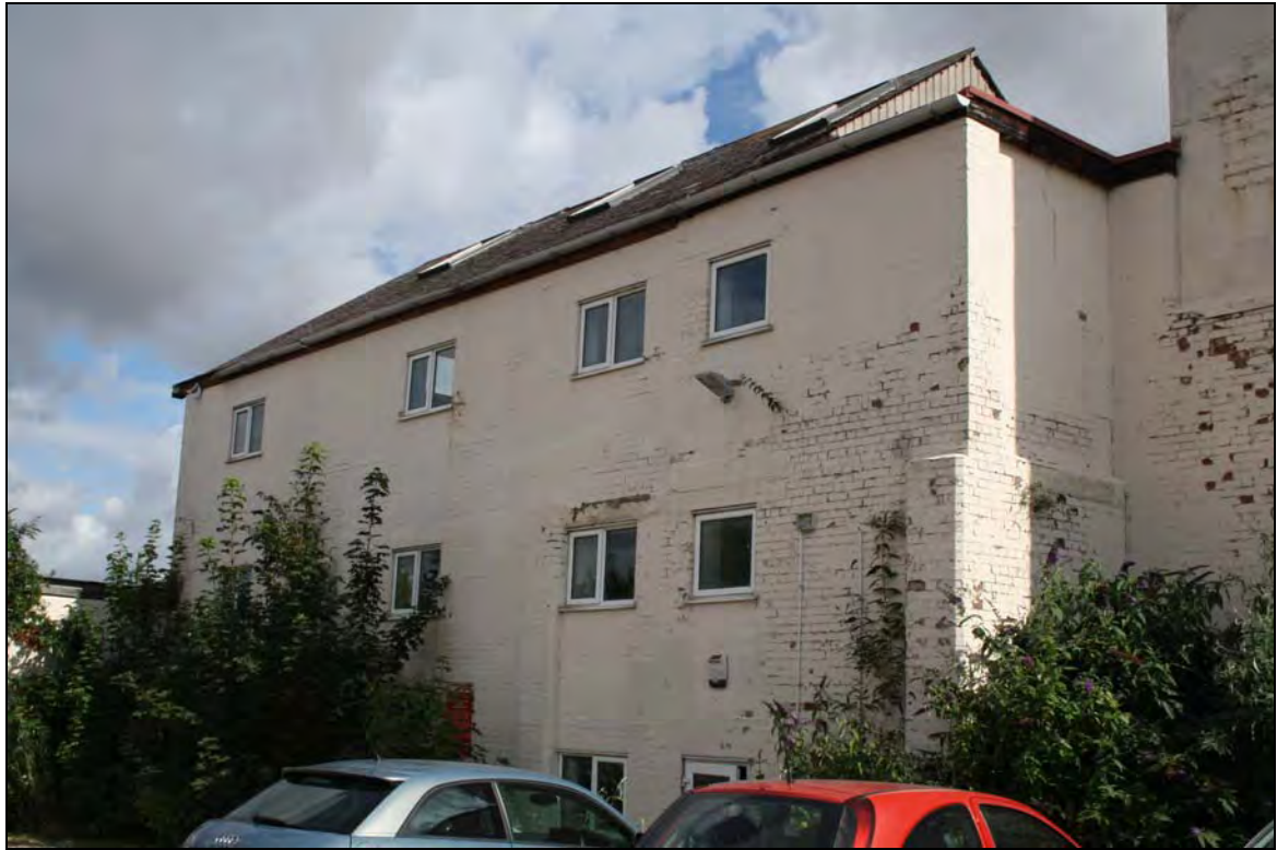
Plate 9 West elevation of Range 3, taken from the south-east (DP 14)
