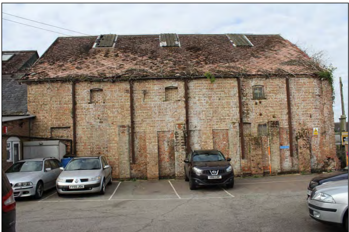
Plate 4 North elevation of Range 1, taken from the north (DP 55)
