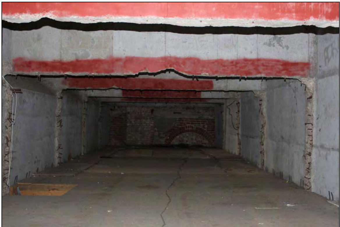
Plate 6 First floor of Range 1 (FF01) showing removed lower concrete structure of the silos, taken from the west (DP 120)
