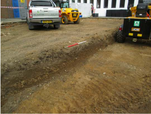
DP 7. South-west part of the excavation area. Looking west.
