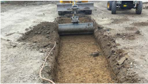
DP 3. Further ground reduction in the central area. Looking south-east.
