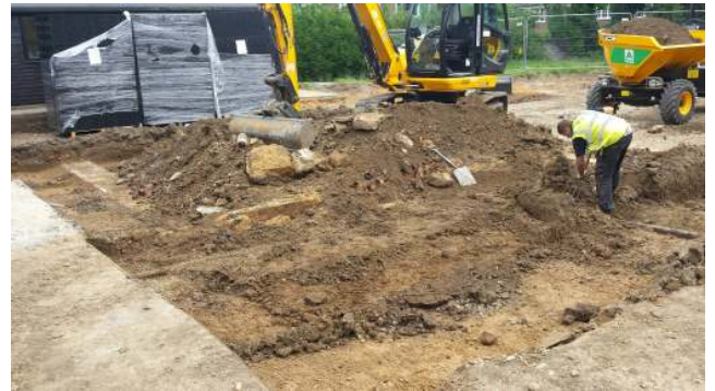
DP 4. Works in the central part of the site. Looking east.
