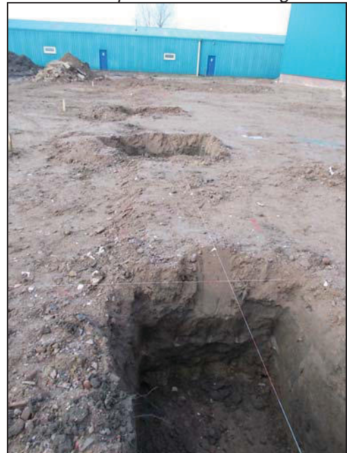
10 View of excavated pads, looking west.
