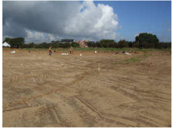
2: Site shot (under excavation), looking N
