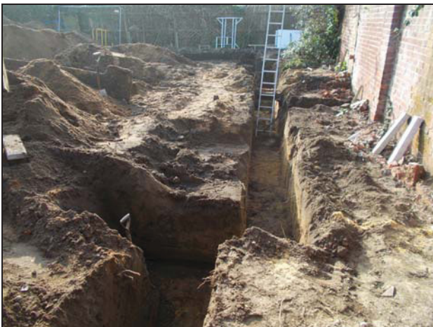
11 View of northernmost footing, looking west.
