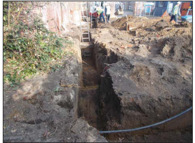
10 View of northernmost footing, looking east.
