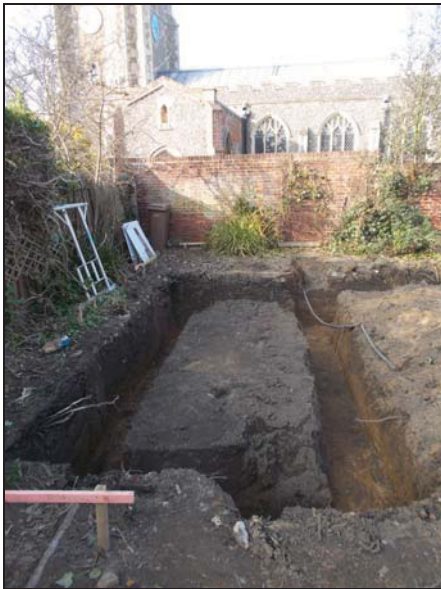
9 View of westernmost footings, looking north.
