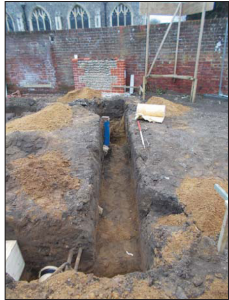
8 View of easternmost footing, looking north.
