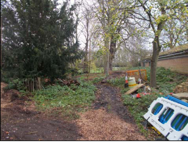
1 Pre-excitation view of site looking north
