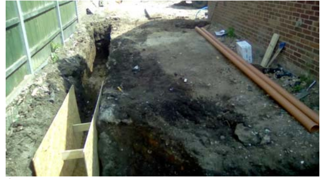
2 Post excavation view of footings looking north-east
