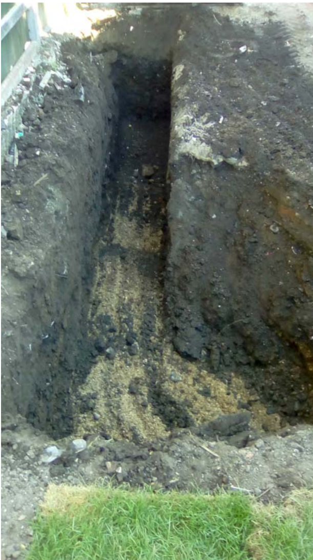
3 View of footings in south-west corner of site
