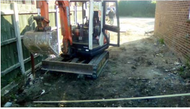
1 General view of site before excavation of footings looking north-east
