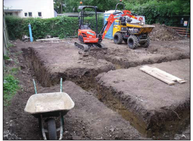
2 General view of footings looking south-west
