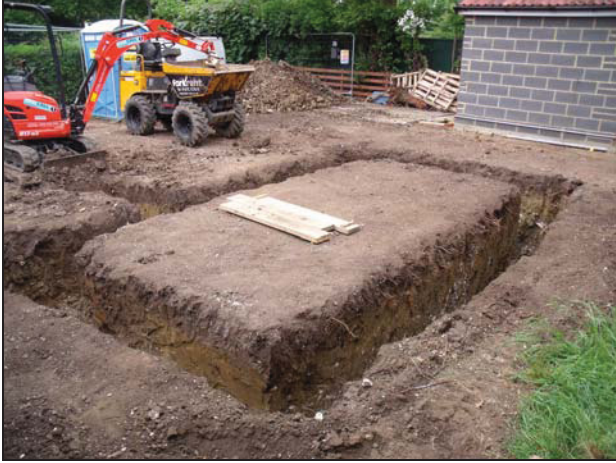
1 General view of footings looking south-west
