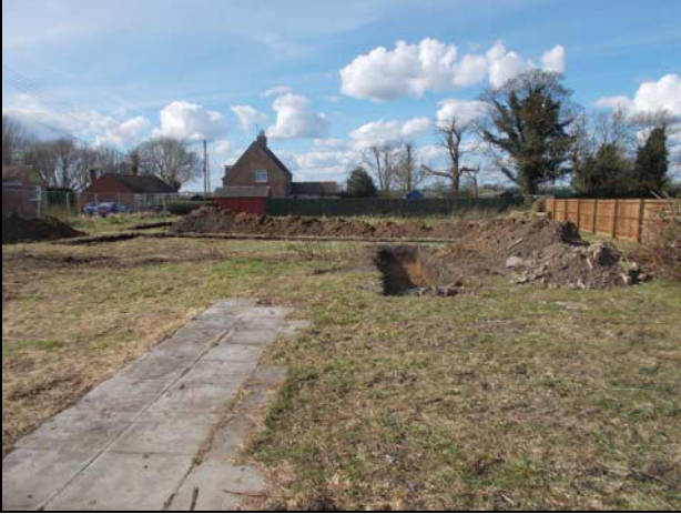
1 General view of excavated trenches
