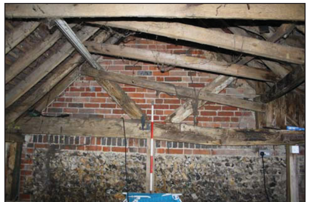
Outbuilding, original external wall of brick and flint element and end truss of timber framed section, taken from the east
