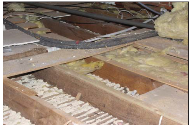
Detail of the floor joists in the roof space following the removal of modern boarding, taken from the south-west
