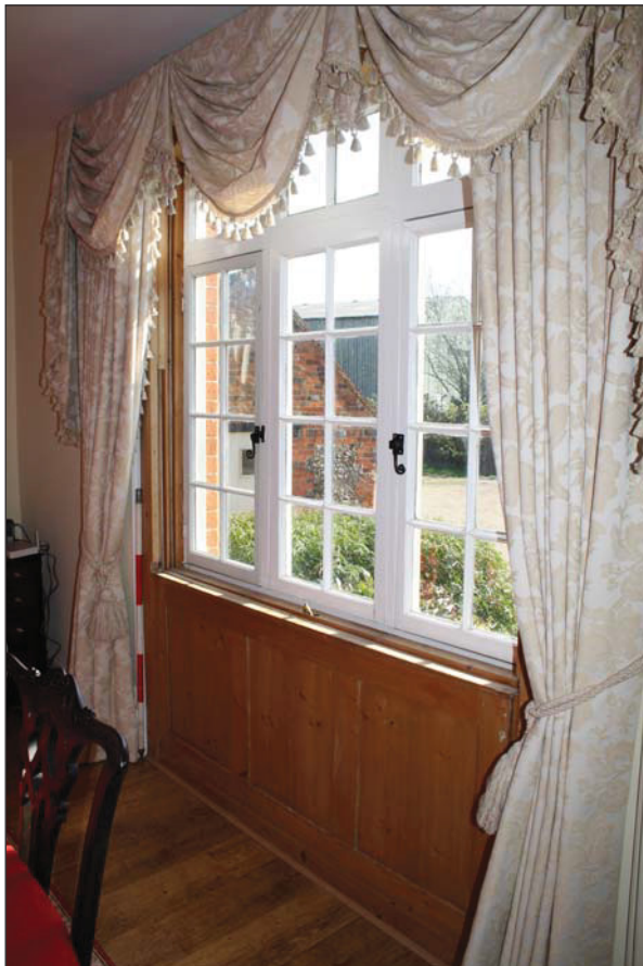
Plate 4 Three-light casement window with shutters, GF02, taken from the north-west (DP 27)
