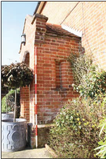
3 Gothic style porch, south elevation, taken from the south-east
