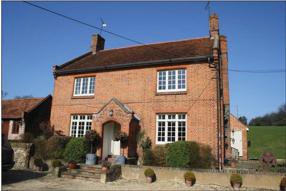
Plate 1 Dane Farmhouse, south elevation, taken from the south-east (DP 1)
