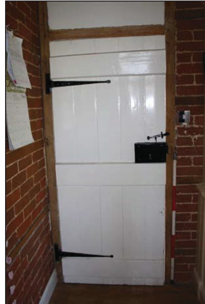
Door with rim lock and strap hinges, GF03, taken from the east
