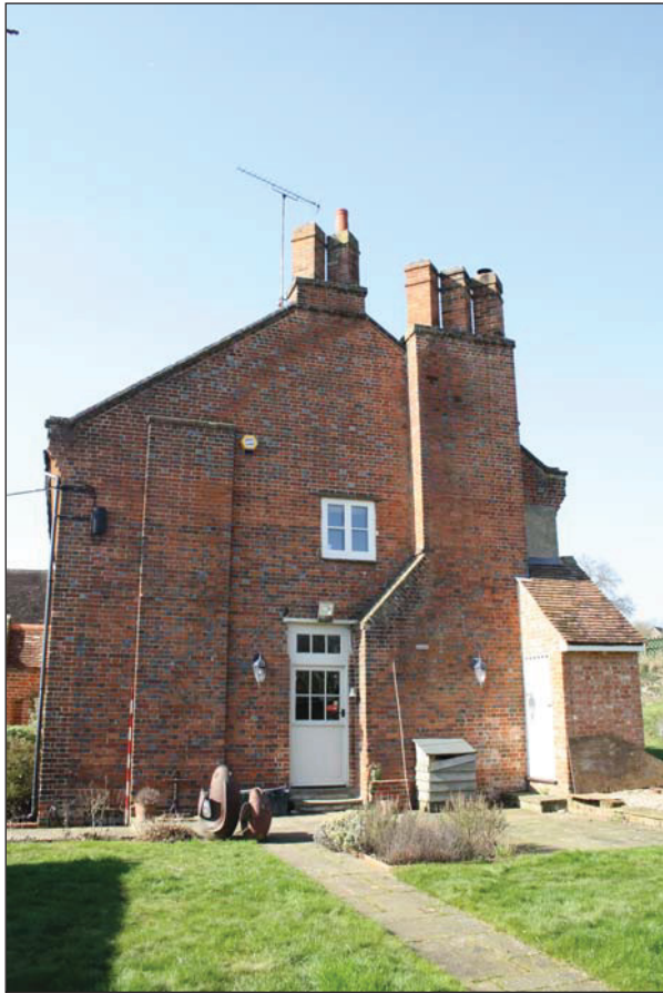
Plate 3 East elevation, taken from the east (DP 5)
