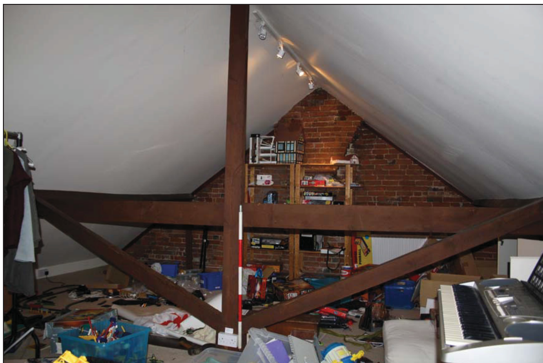
Plate 8 King post roof truss, attic, taken from the north-east (DP 41)
