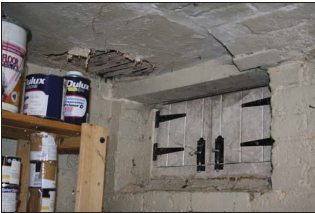
Re-used timber above the window in GF03, taken from the south-west
