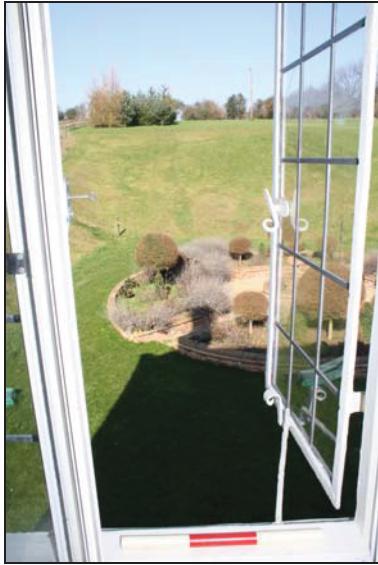
31 Window with hook stay and handles, FF01, taken from the south from the south
