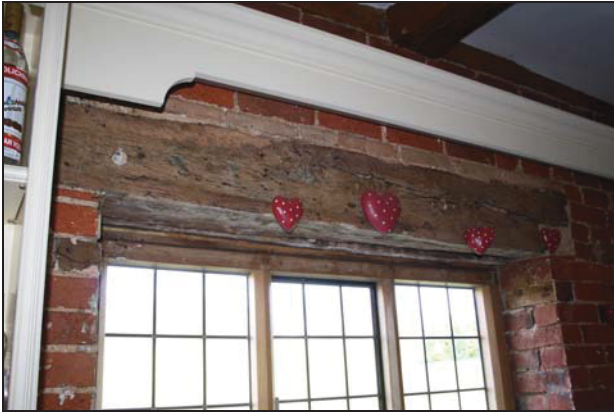
Re-used timber above the window in GF03, taken from the south-west
