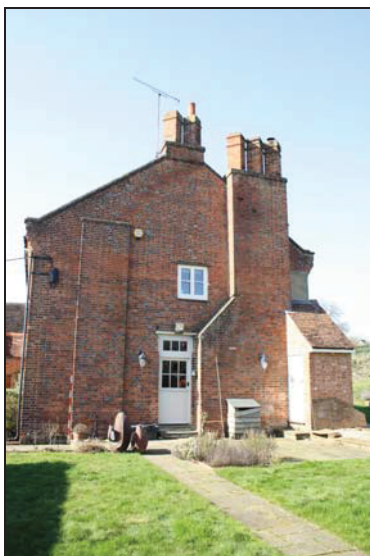
5 East elevation, taken from the east
