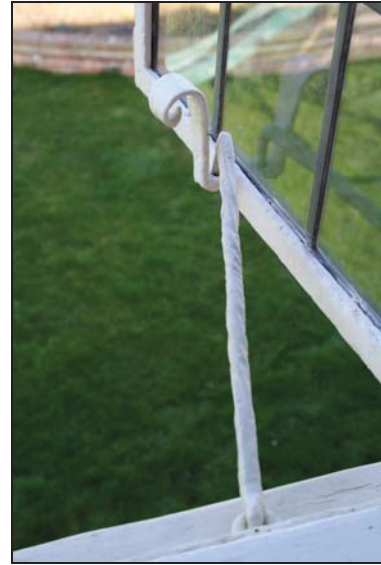
32 Window with hook stay, FF01, taken from the south
