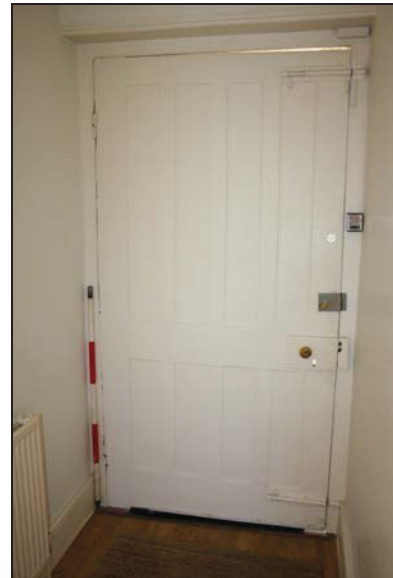
Door with rim lock and strap hinges, GF03, taken from the east
