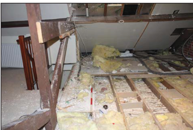
View of the floor joists in the roof space following removal of the modern enclosed closet, taken from the south
