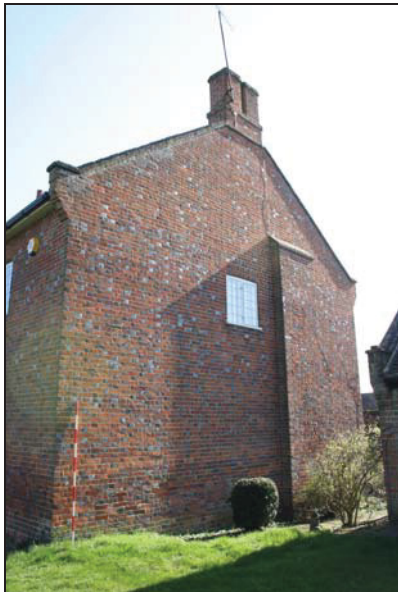
Cellar light with gauged arch, east elevation, taken from the south-east
