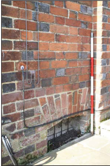
Cellar light with gauged arch, east elevation, taken from the south-east
