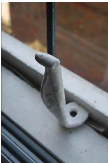
35 Casement handle, FF02, taken from the north-east
