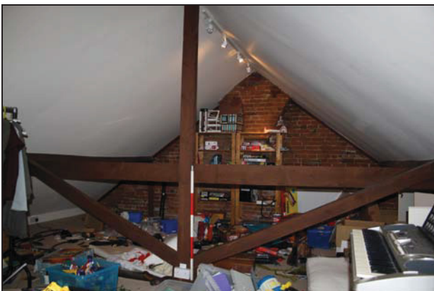
King post roof truss, attic, taken from the north-east
